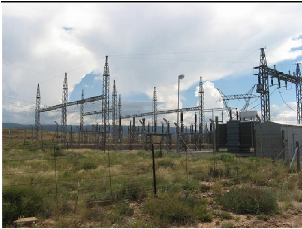
Figure 1.10 Existing Drennan Traction Substation
