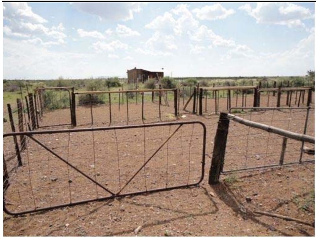
Figure 1.13 View of Derelict Labourers Cottage and Animal Pens
