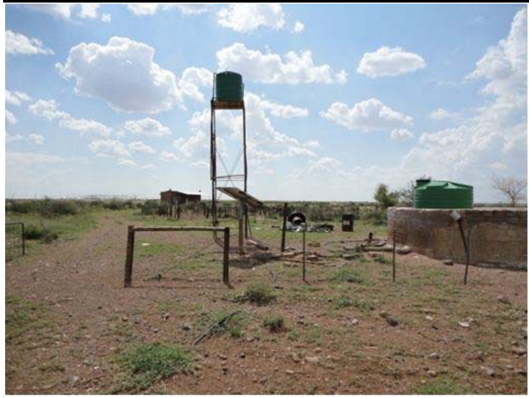
Figure 1.12 View of Existing Borehole on Site
