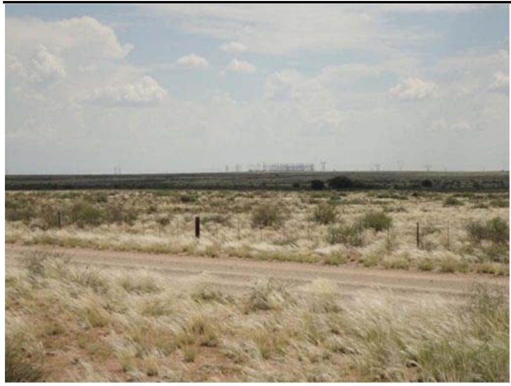
Figure 1.3 Typical Vegetation of the Site with Eskom's Aries Substation and Power Lines
