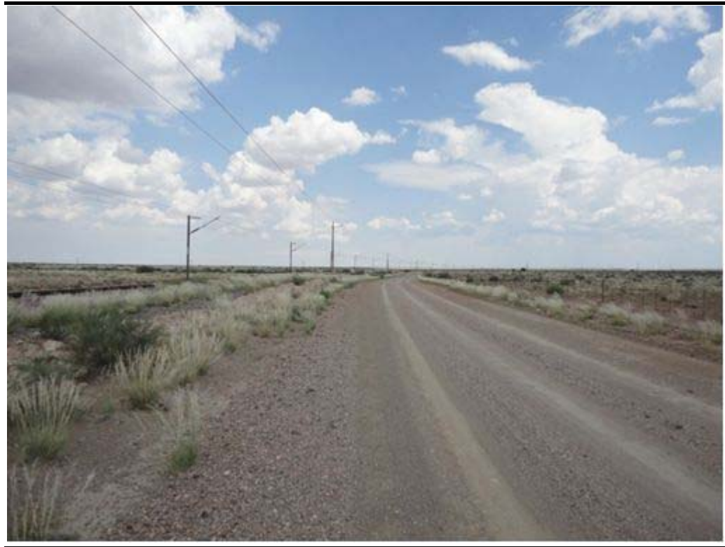
Figure 1.5 View of Sishen- Saldanha Railway Line and Service Road
