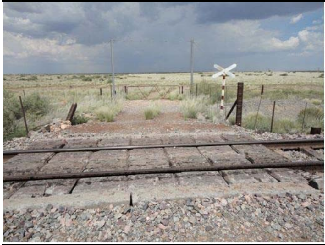
Figure 1.7 Railway Crossing Connecting Two Sections of Olyven Kolk Solar Power Plant Site
