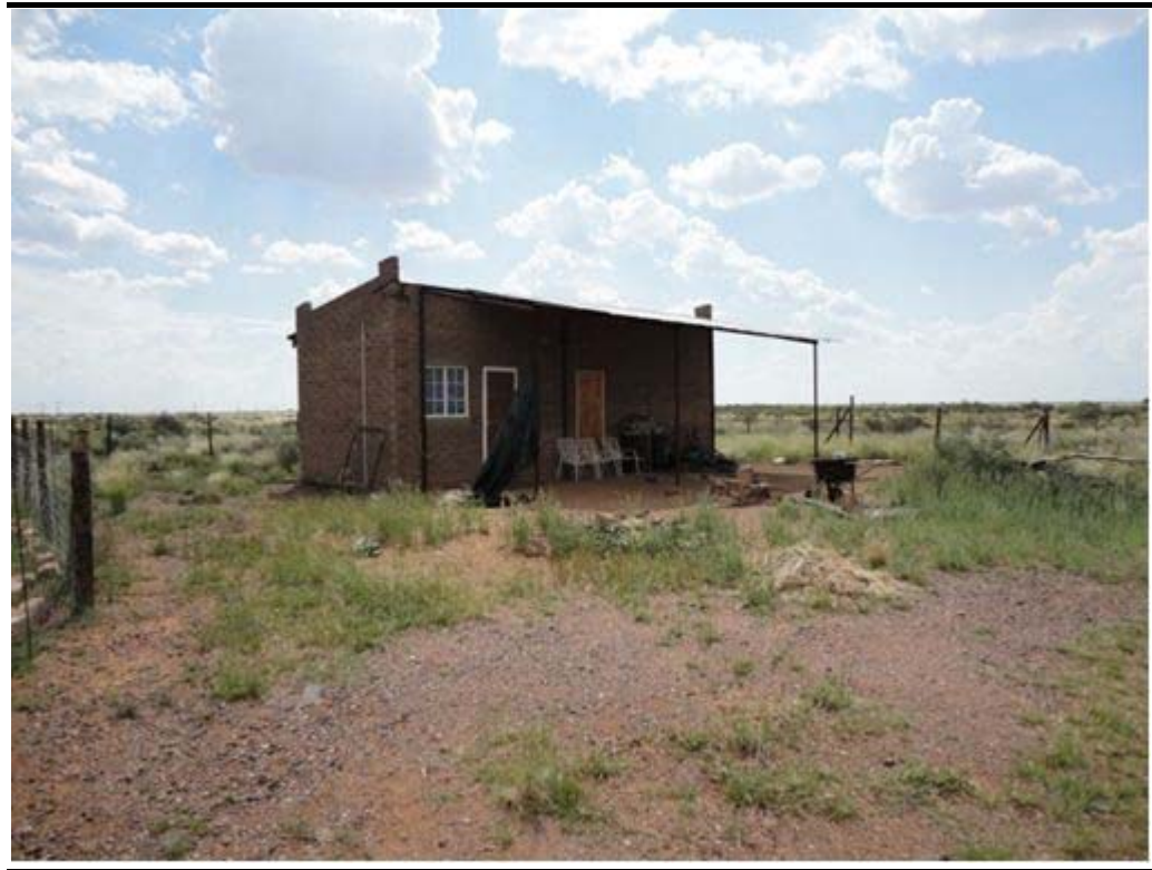
Figure 1.11 Existing Labourers Cottage on Olyven Kolk Site
