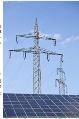
Figure 4: Power lines and PV panels
