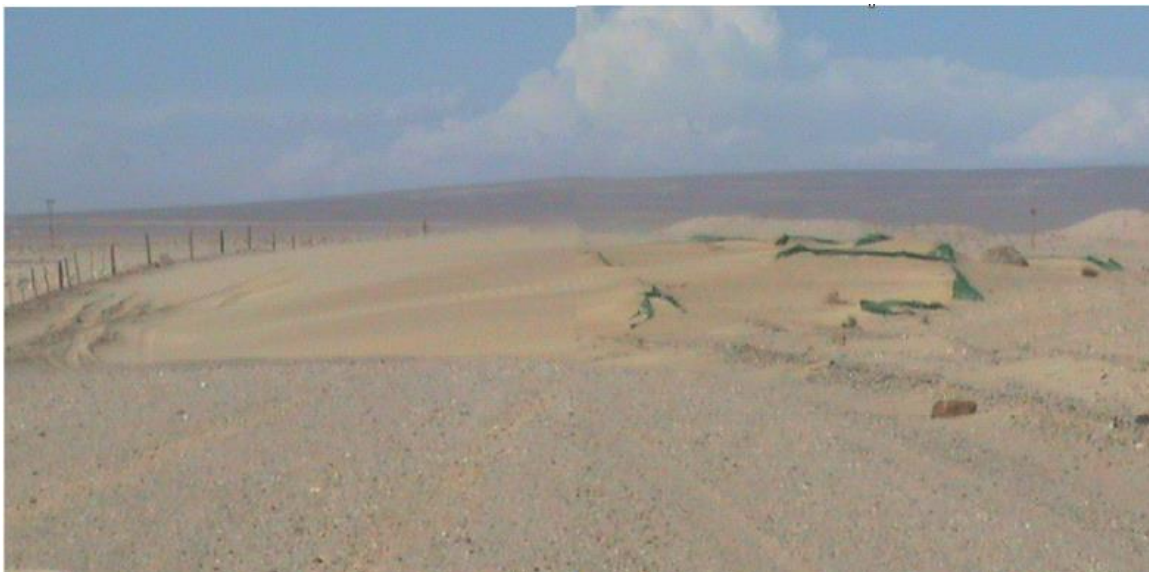
Photo 15: Shows the failure of unmaintained cut-off netting systems at Alexkor at the time
