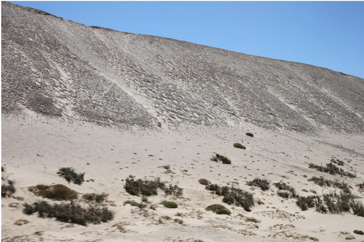
Photo 16: Armouring by coarse tailings of sandy slimes dam wall dust source at Alexkor
