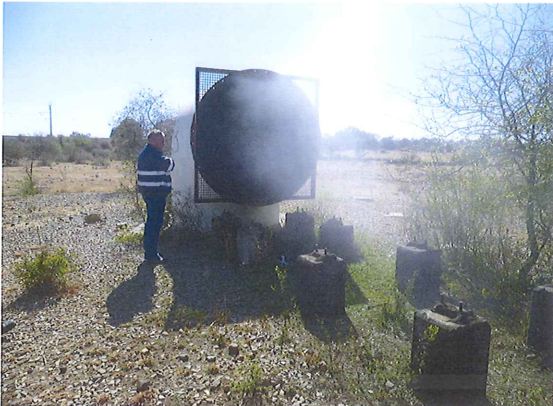
Abandoned Vent shaft in Kanana.
