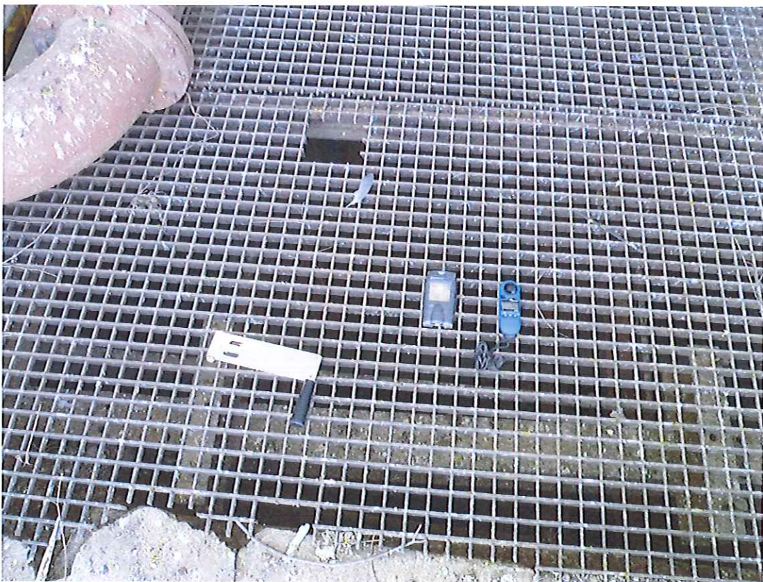
Tests being conducted over the shaft on 6 Shaft Bank.
