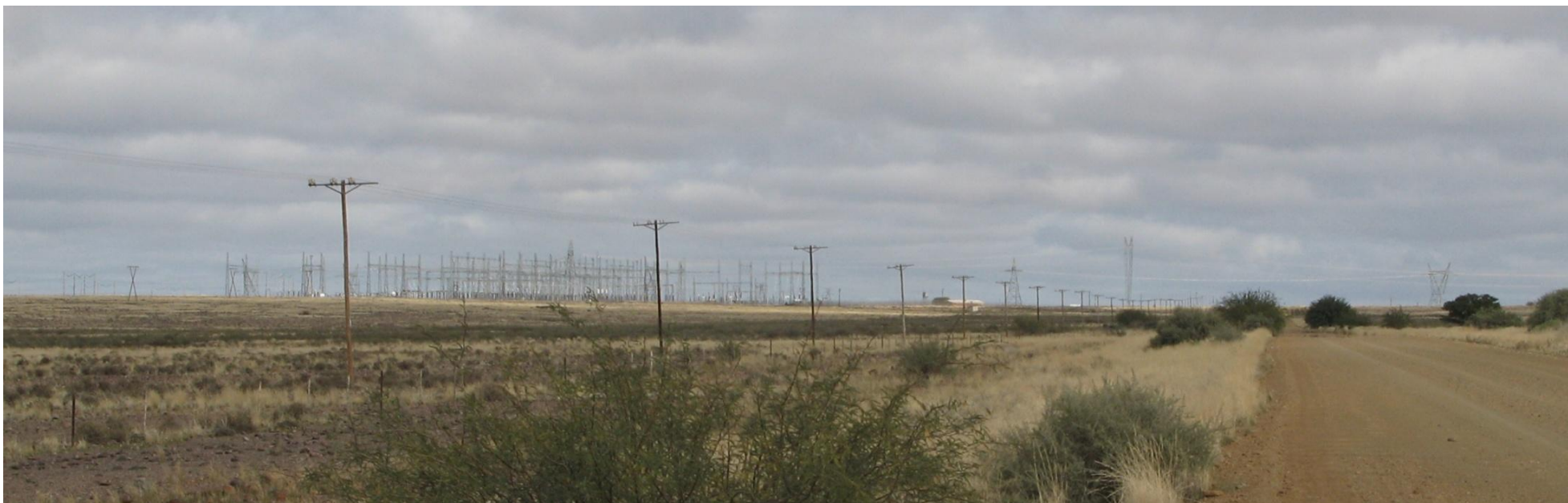
Figure 1: Gravel road sense of place at location with the Aries Substation dominating the landscape context.
