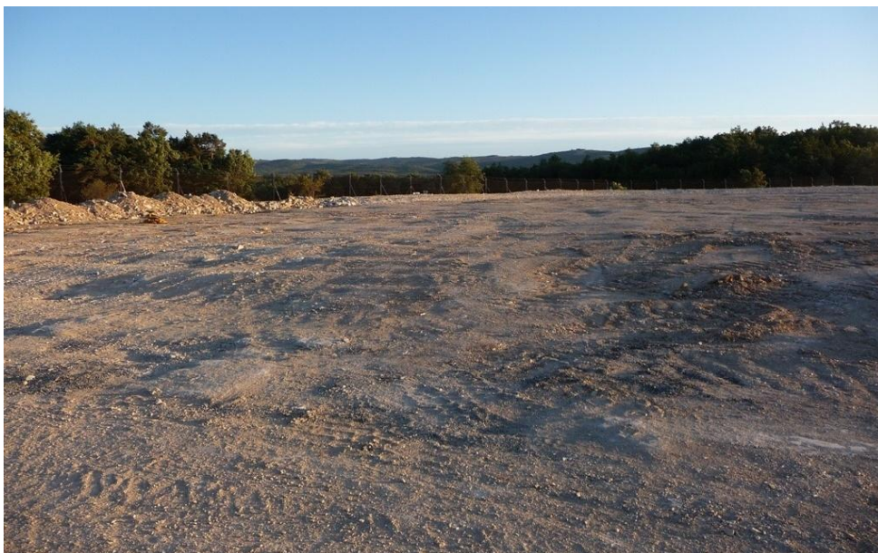
Figure 2: Example of site clearing (Source: ERM)
