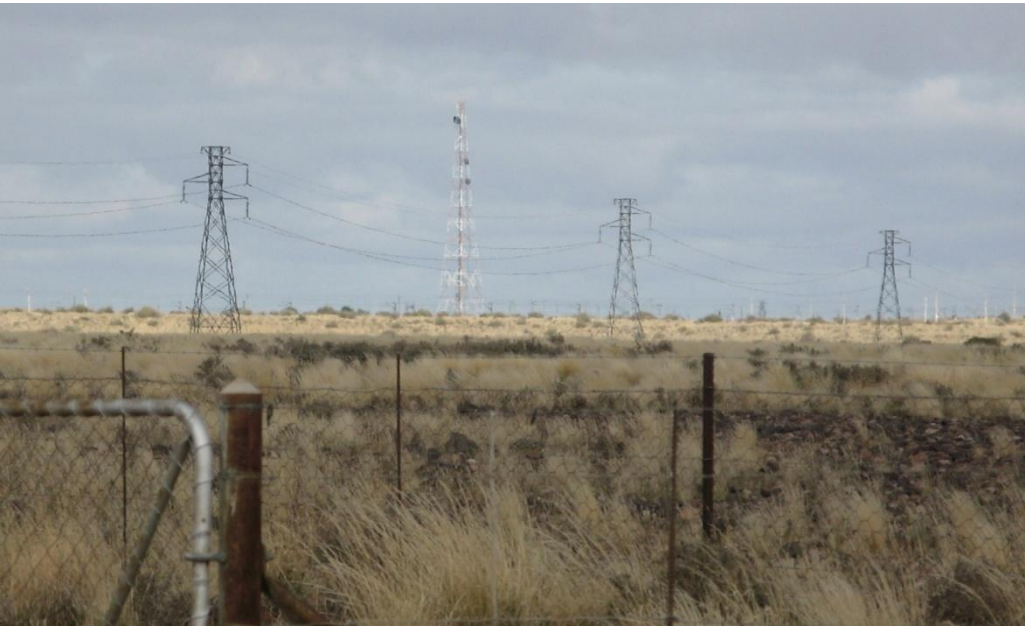
Figure 2: Existing industrial infrastructure (GPS 14)
