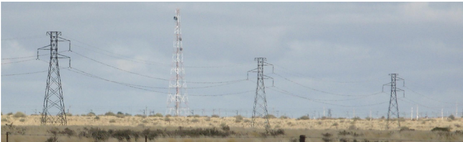
Figure 1: Photograph example of existing power lines in the area (Source: ERM)
