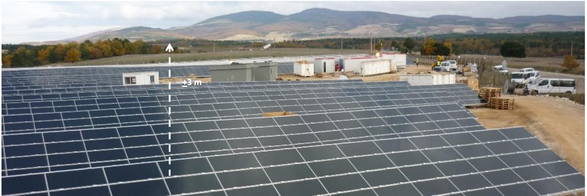
Figure 1: Photograph example of construction site of solar power panels (Source: ERM)
