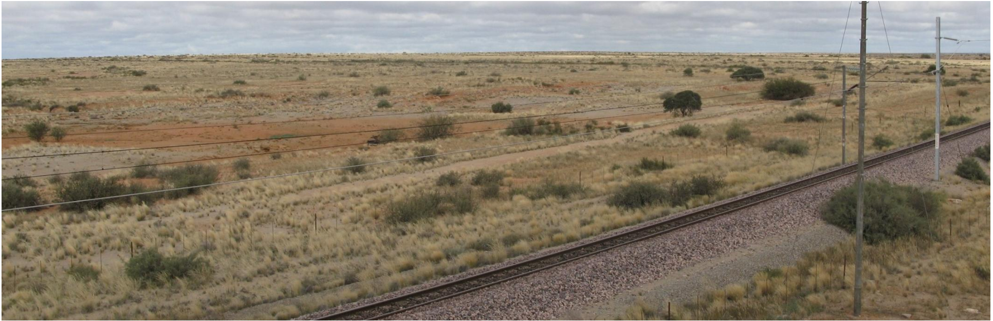
Figure 1: View of existing railway line (GPS 009)
