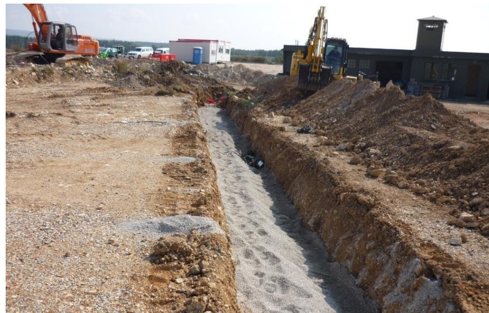
Figure 3: Example trench construction (Source: ERM)
