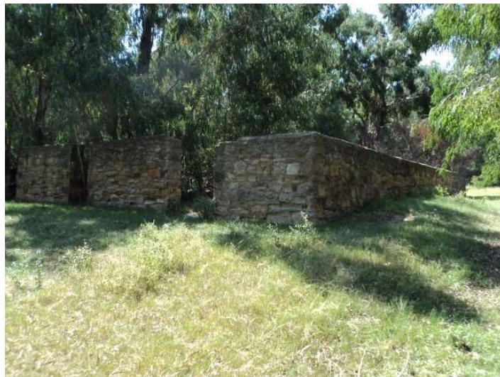
Figure 17: Example of a dilapidated historical kraal.
