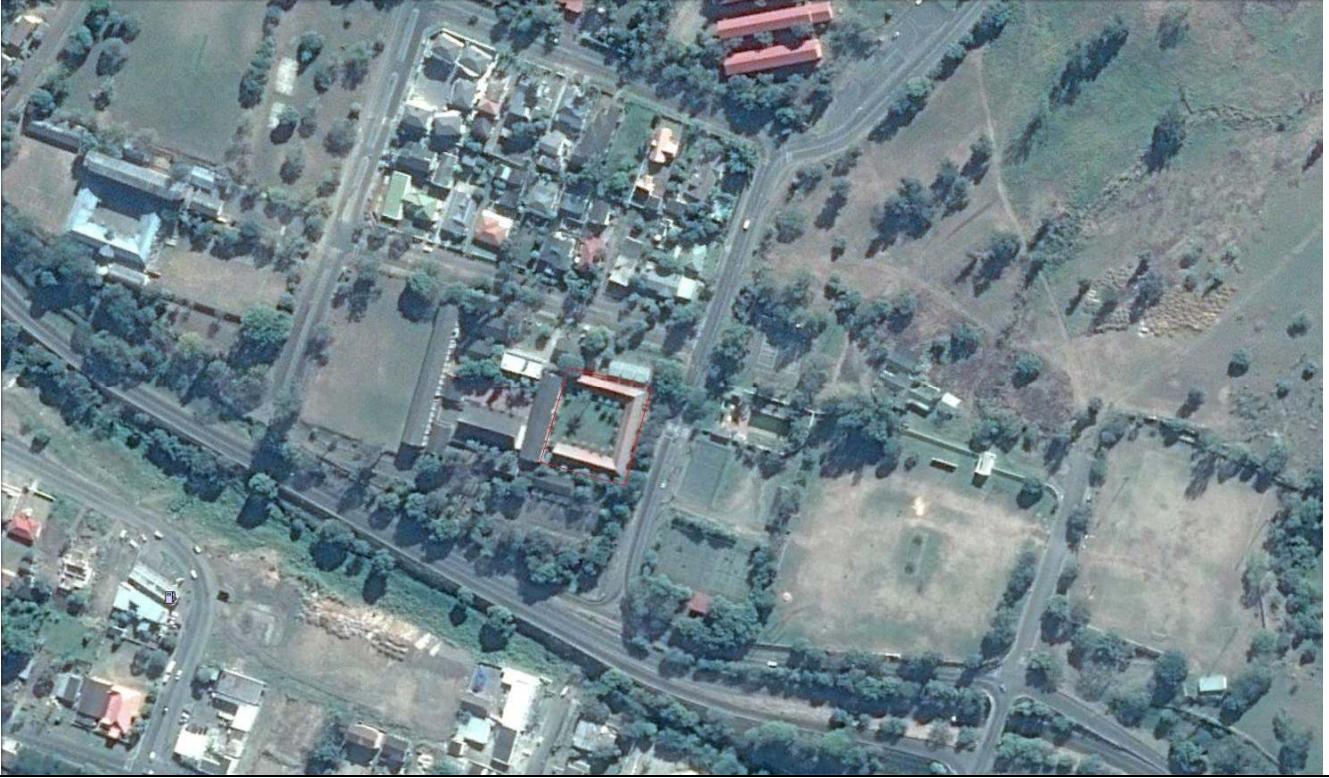
Image 22 – Google map block C: Aerial shot showing how building fits in to the surrounding area
