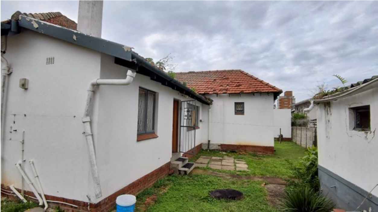
Figure 10. South West Elevation of Main Dwelling with outbuilding on the right hand side. Additions from 1981 were undertaken to this facade and are visible due to the ad hoc manner in which it was undertaken.
