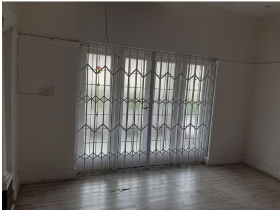
Figure 21. Internal view of lounge area. Painted timber suspended floors. Picture rails
