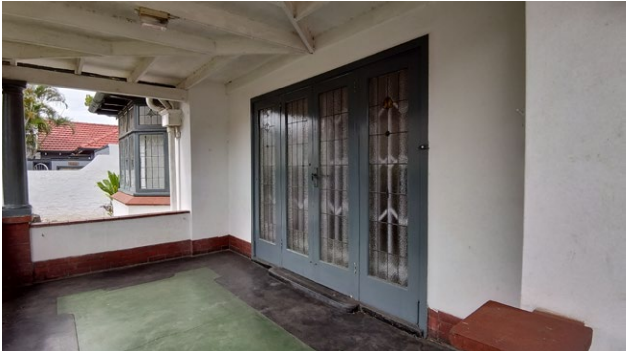
Figure 8. View of entrance verandah. Verandah consists of black and green stoep paint.
