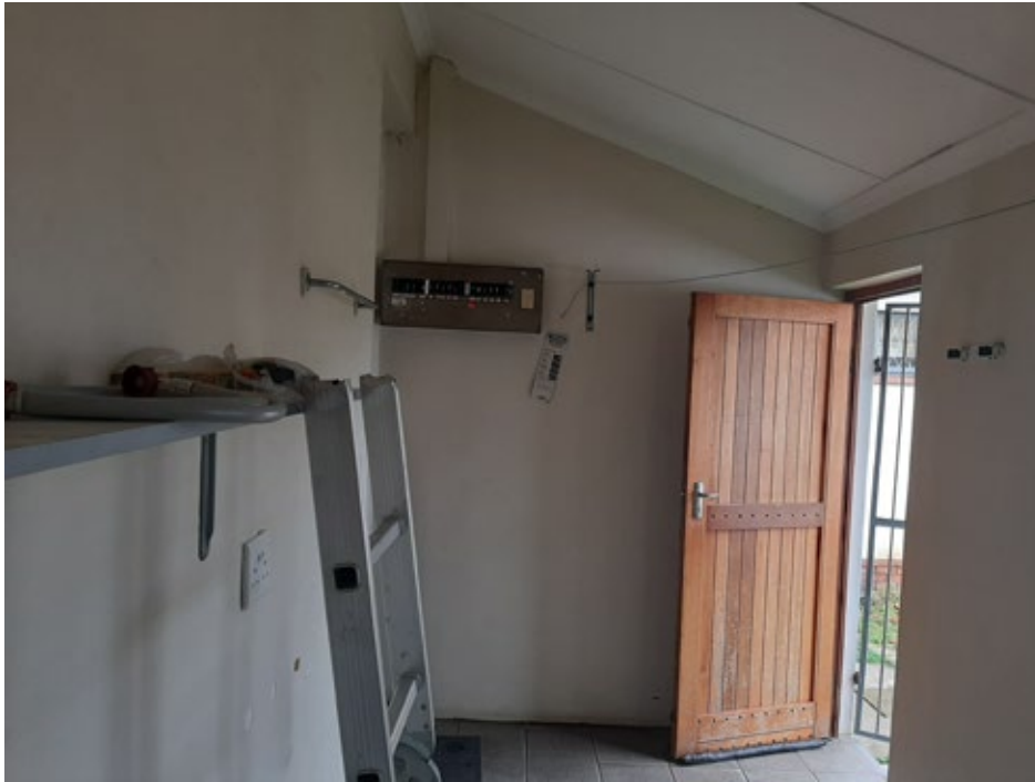
Figure 19. Internal view of laundry room
