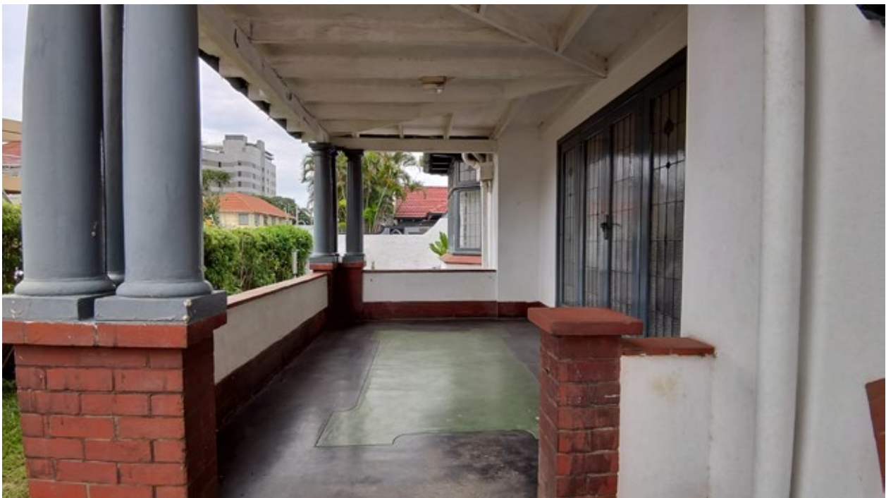
Figure 7. View of entrance verandah. Verandah consists of black and green stoep paint.
