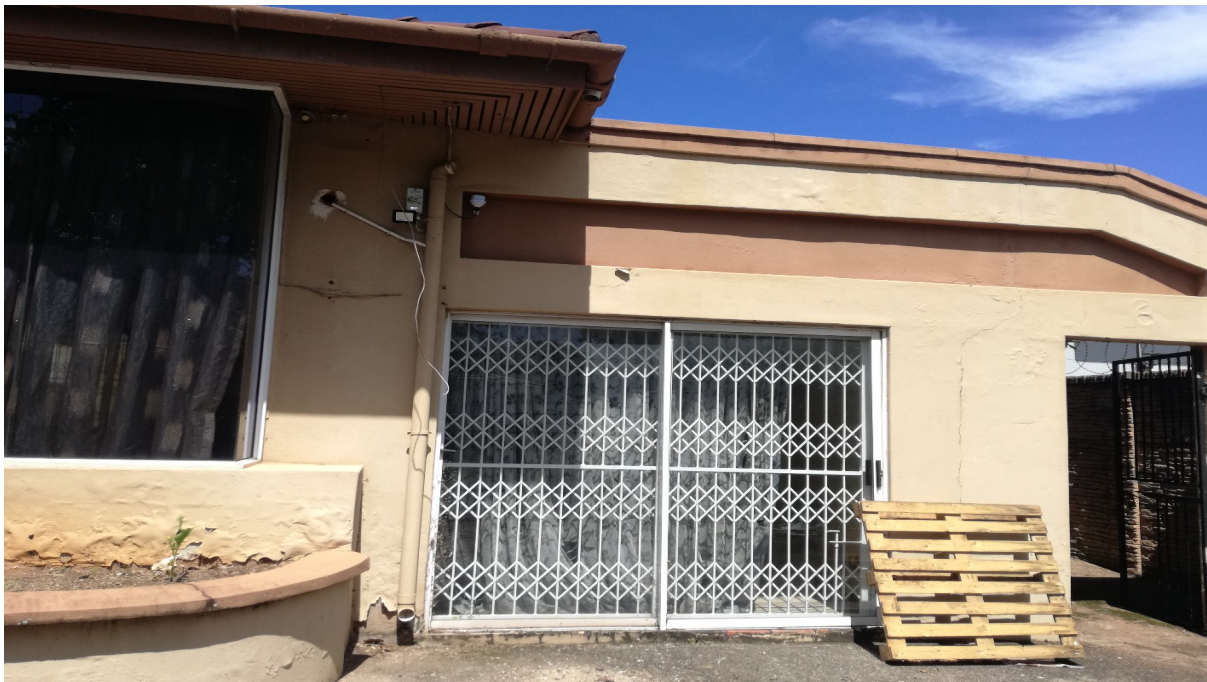
Figure 8. View of verandah front door
