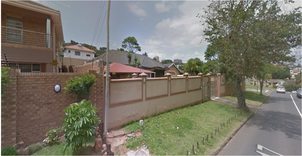
Figure 1. Street View (Hendry Road)
