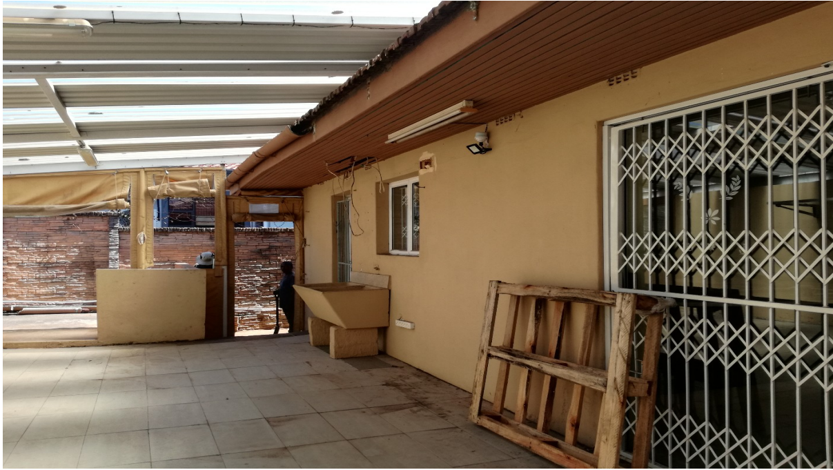
Figure 5. Rear elevation view of house from covered back yard
