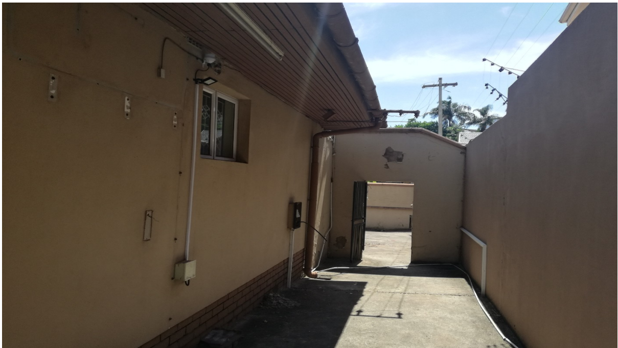
Figure 4. Side elevation view of house from garden
