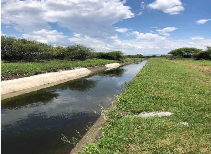
Concrete canal within the site
