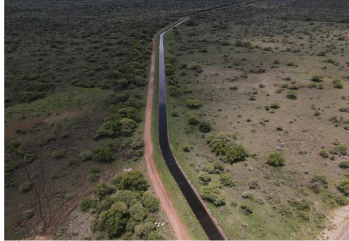
Aerial view of the canal
