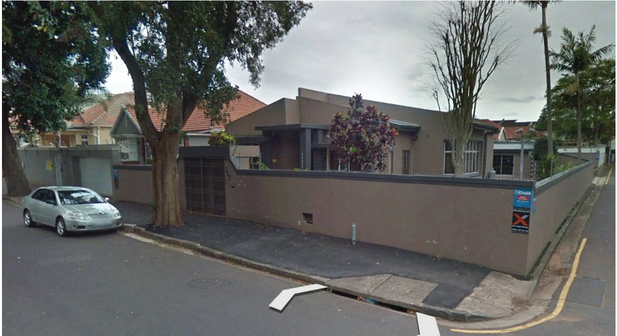
Figure 1. 268 STEPHEN DLAMINI ROAD - EXISTING HOUSE
