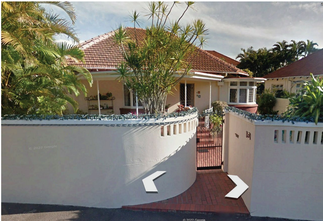
Figure 12. 19 CAISTER CRESCENT - EXISTING HOUSE USED AS OFFICE
