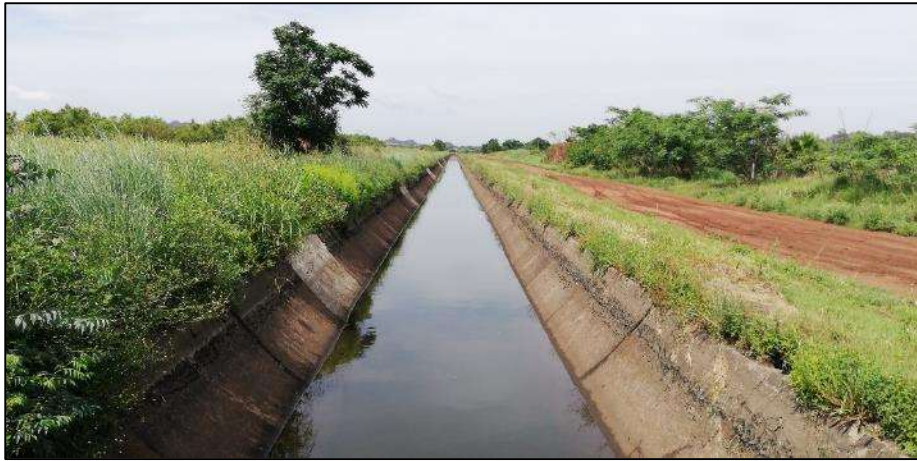
Figure 5: Canal associated with RE/14/420.
