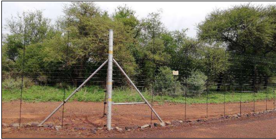
Figure 9: Fenced-off section on 845/420.
