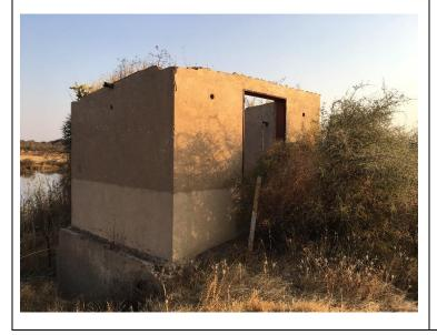
An old pump-house constructed in the past located on the bank of the Vaal River. It is expected that this structure will be used to house the future pump to limit additional impacts on the bank of the river.
