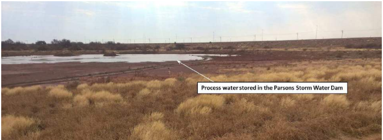
FIGURE 5: WATER CONTAINED IN THE PARSONS STORM WATER DAM
