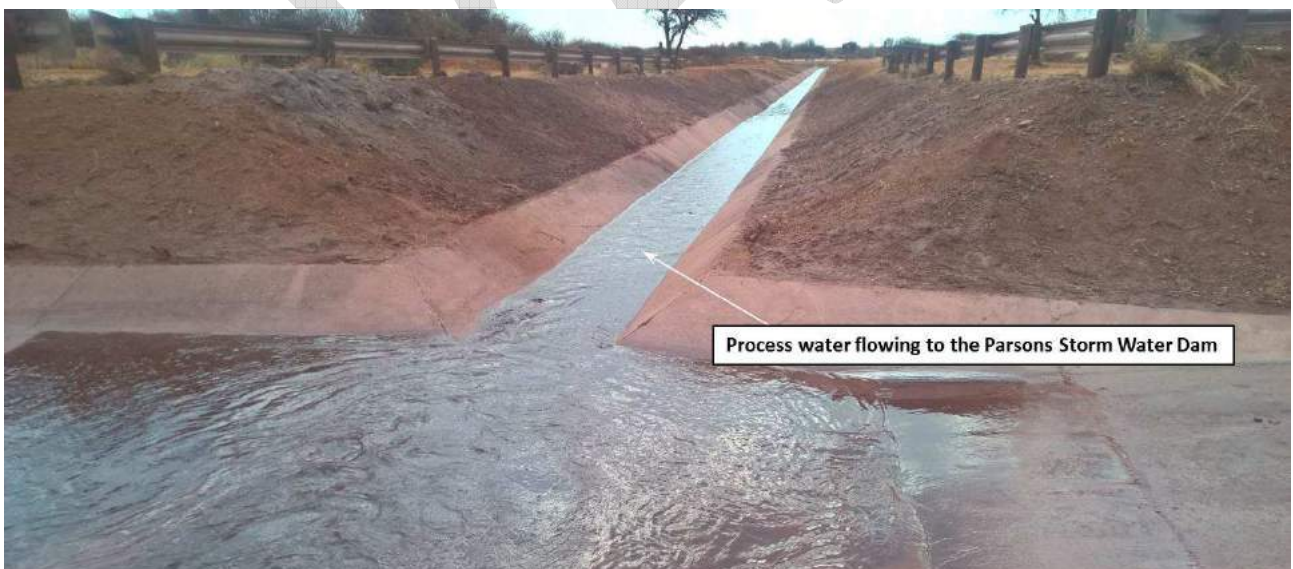
FIGURE 4: WATER REGULARLY FLOWS DOWN THE TRENCHES TOWARDS THE PARSONS STORM WATER DAM
