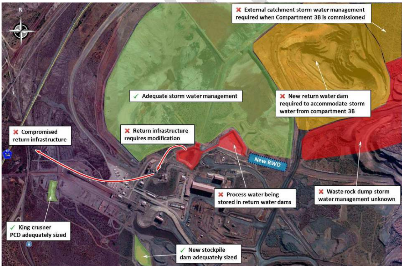
FIGURE 6: SUMMARY OF THE KING STORM WATER MANAGEMENT AND GN 704 COMPLIANCE FINDINGS
