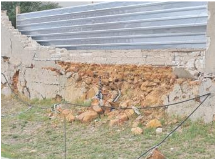
Fig 6. View of the northern wall showing temporary security measures. 2022.
