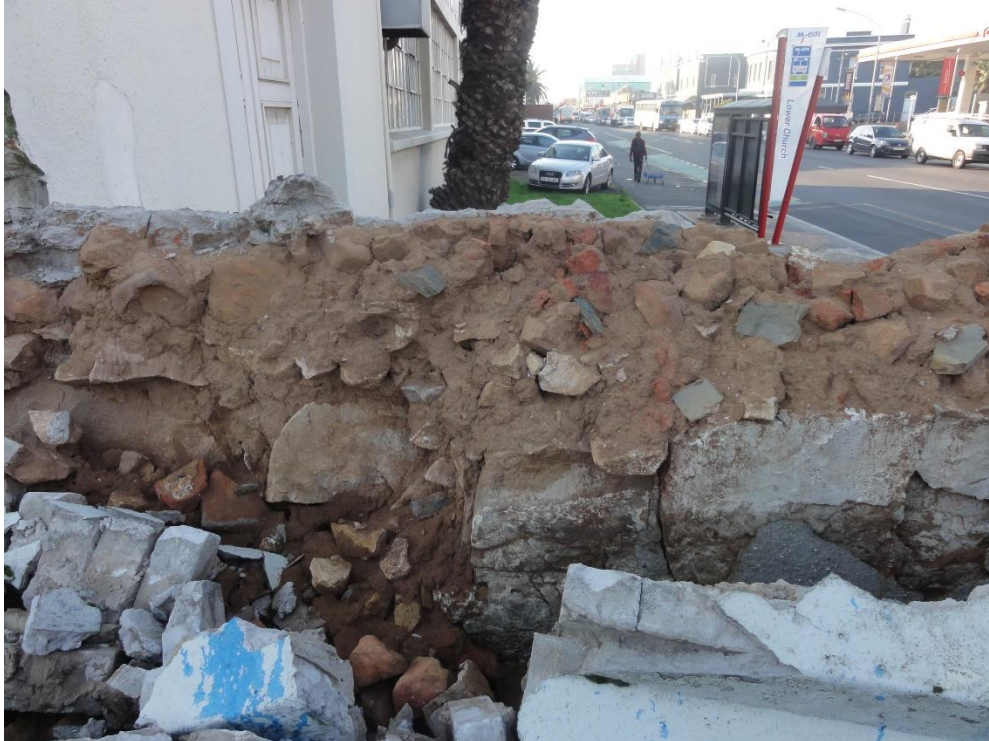
Fig 4. View of the eastern wall looking along Albert Road photo 2018.
