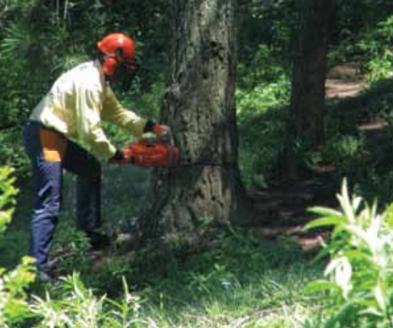
Above: Chainsaw operator felling a Pine tree.
