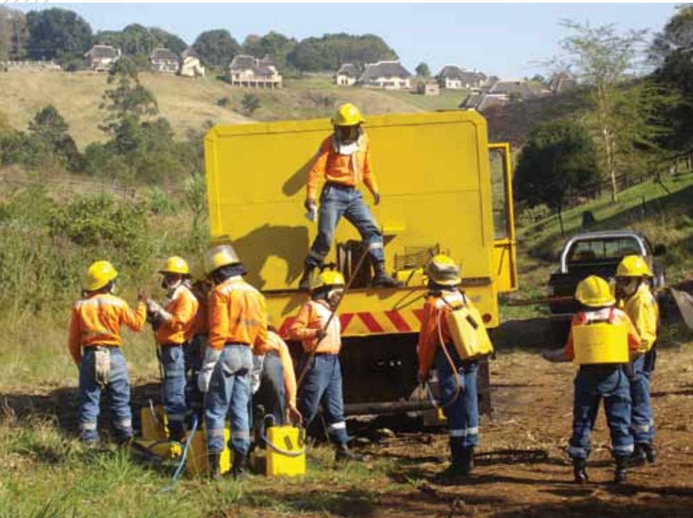
Above: Team of workers in safety gear ready to start clearing.
