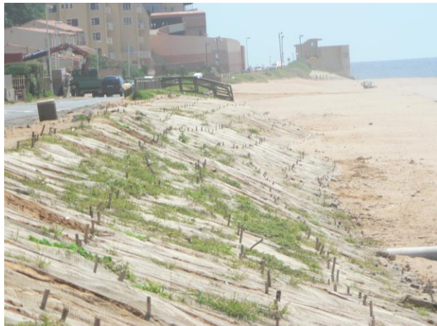
Figure 10: Geo-textiles together with indigenous dune vegetation used to stabilise coastal embankment along Durban's coastline.
