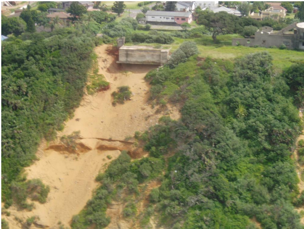
Figure 2: Damaged dunes along Durban's coastline.
