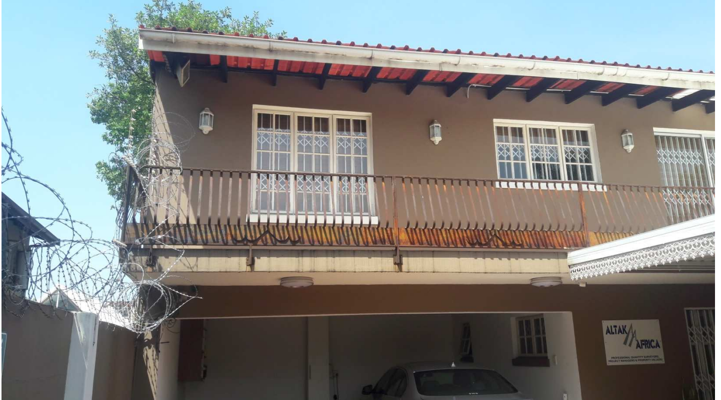
View of added outbuilding (garage and office).
