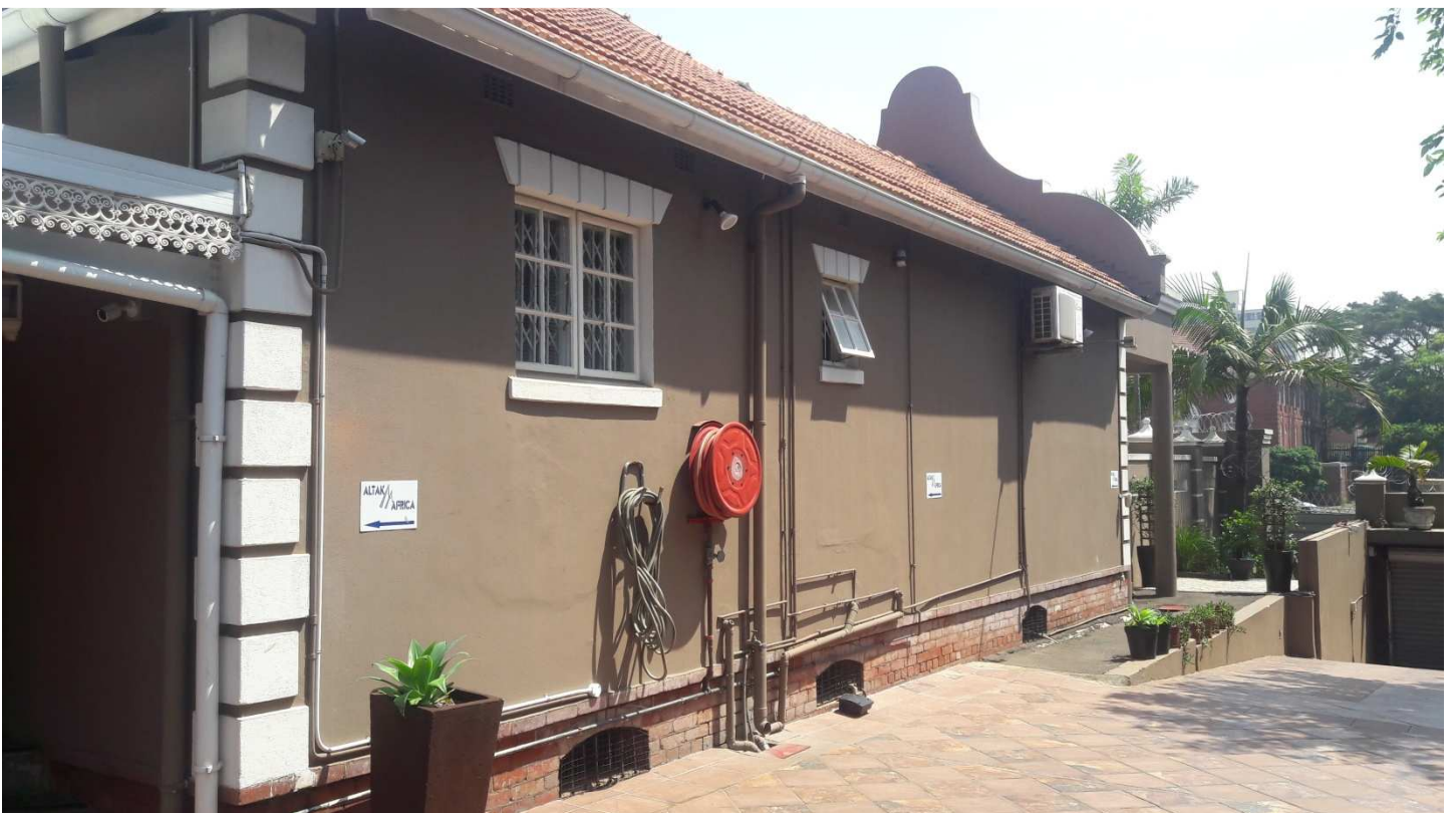
SE view of existing dwelling with added carport to the left.
