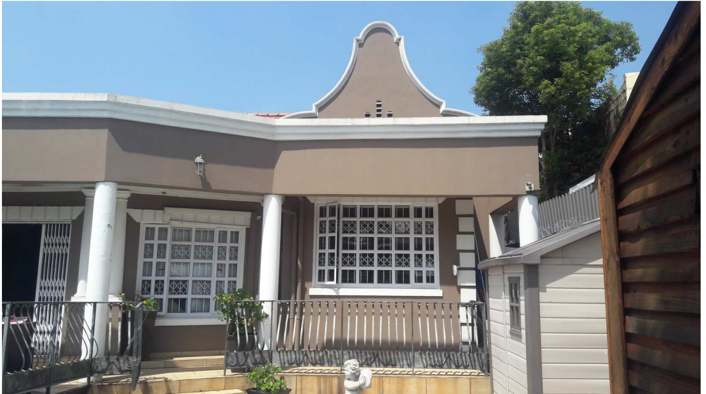
NE view of existing dwelling.
