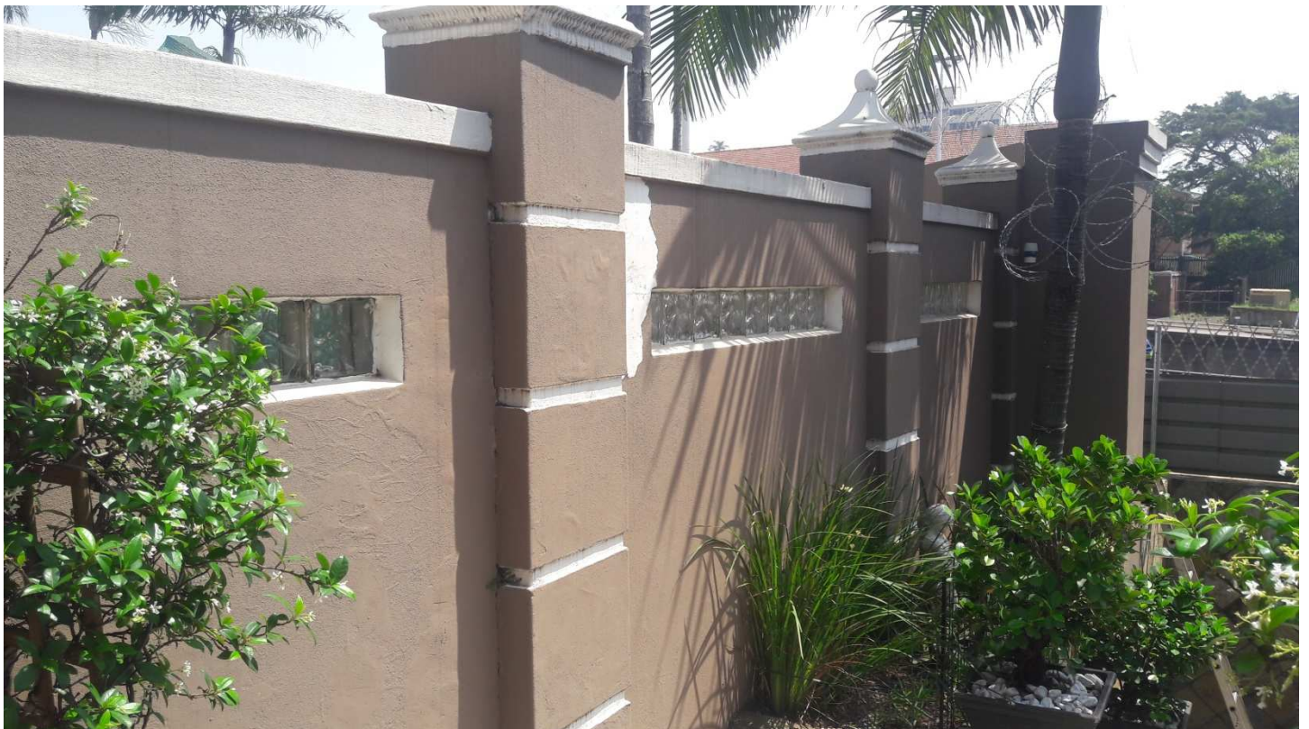
View of added boundary wall (street front) from inside the property.
