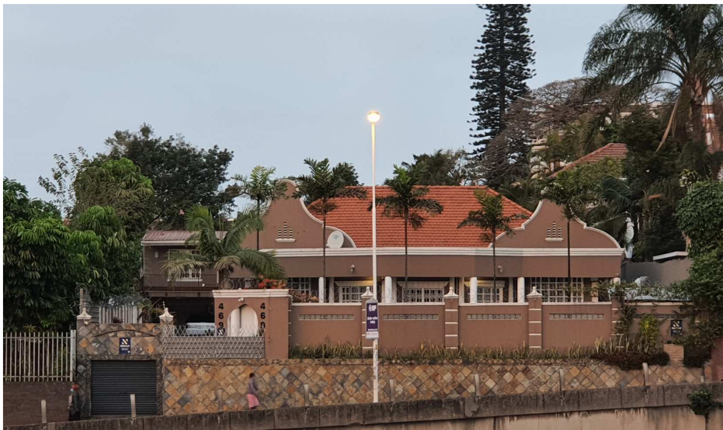
View from across the street - added colonnade, outbuilding in background and boundary wall.
