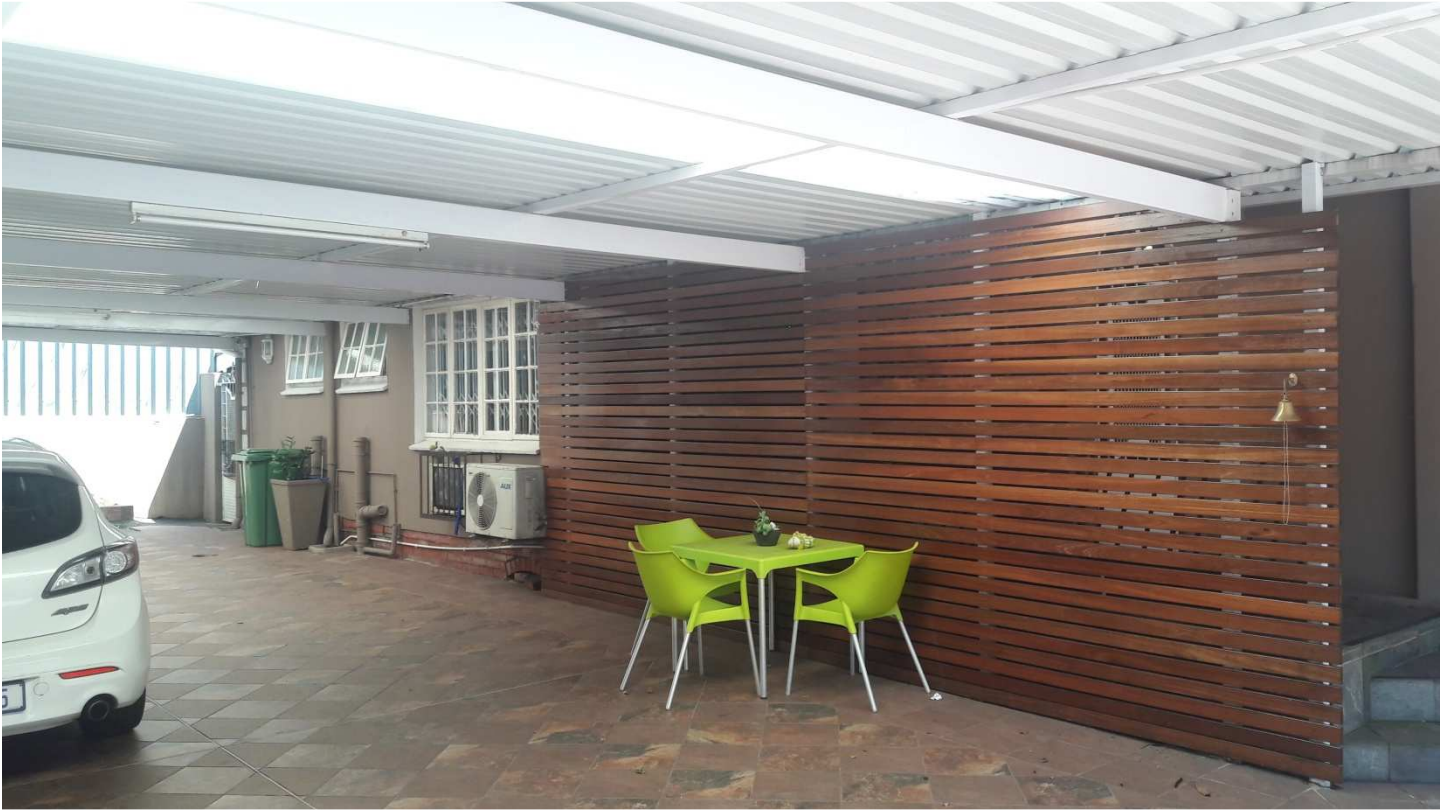
SW view of existing dwelling with added carport overhead.
