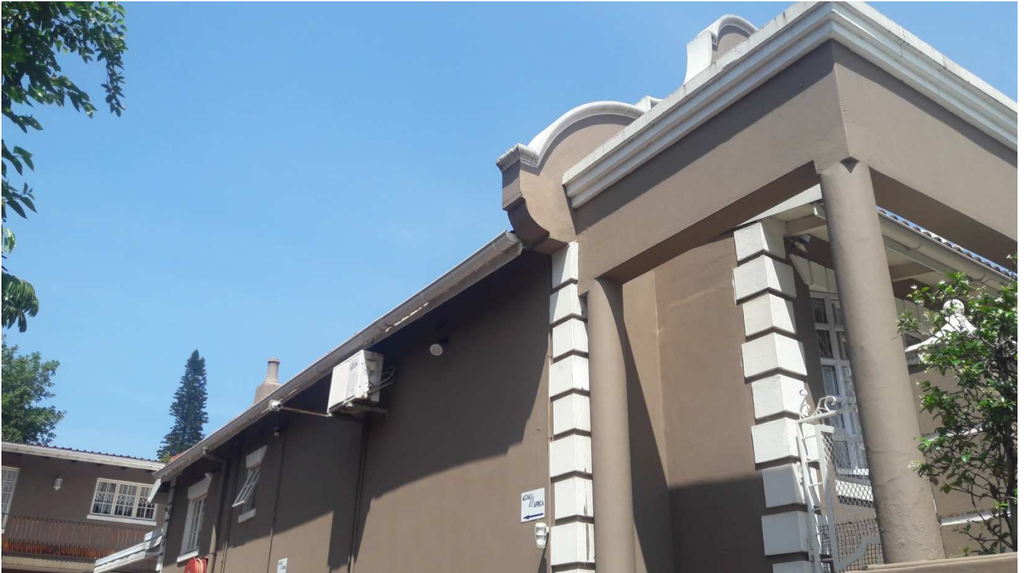
SE view of existing dwelling, with added outbuilding in background..
