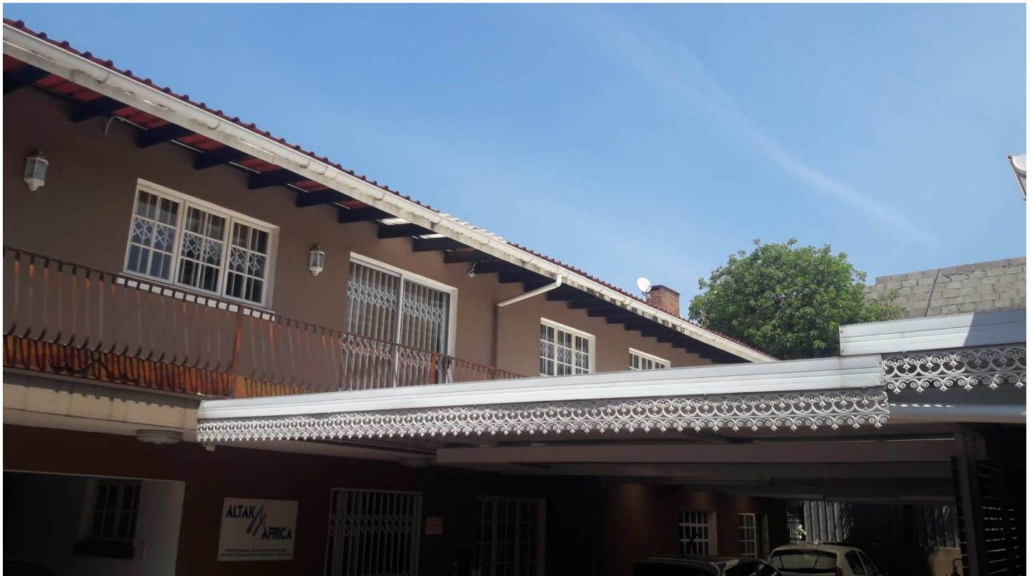
View of added outbuilding (garage and office) and carport.
