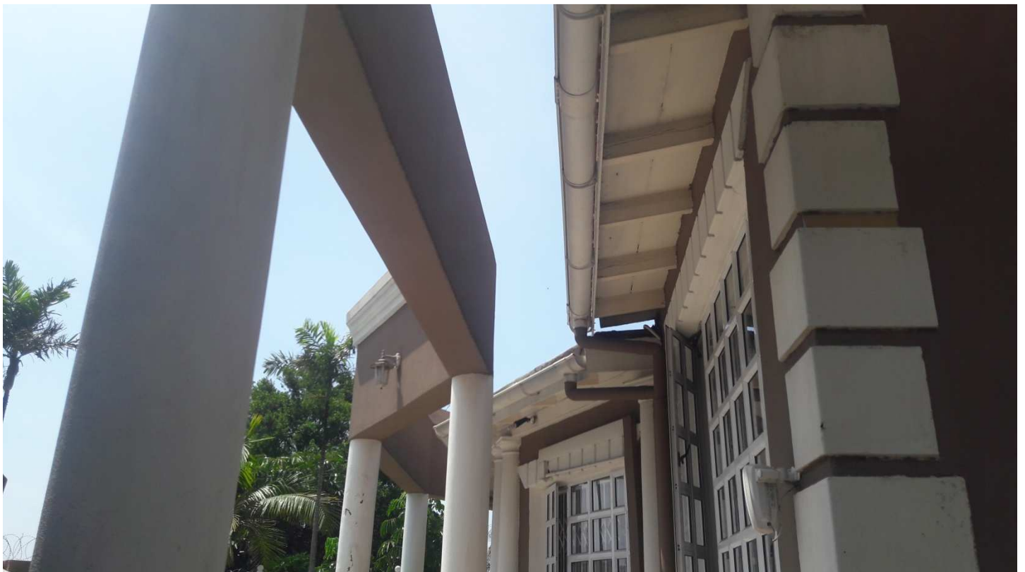
Close-up view of added colonnade.
