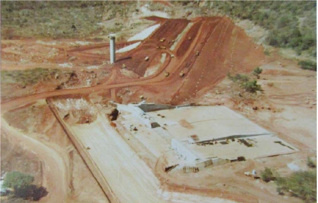
Figure 3: Embankment zoning during construction
