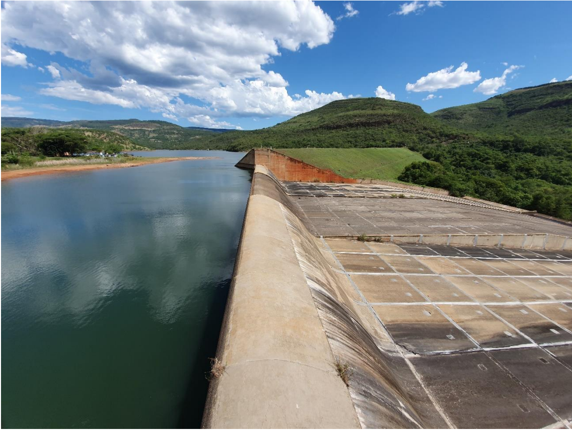
Photo 1: General view of spillway and dam embankment from right flank (19 November 2019).
