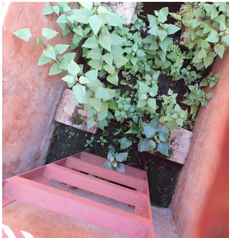
Photo 12: V-notch weirs in chamber at embankment toe to measure seepage flow from sub-soil drains (19 November 2019). Note overgrown state and sediment which will influence accuracy of readings.
