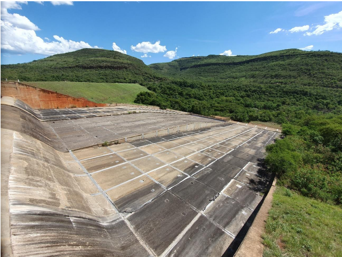
Photo 2: Spillway discharge channel looking downstream from right flank (19 November 2019).
