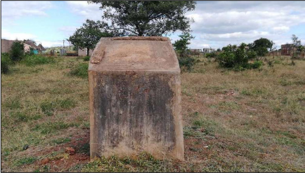
Figure 31: Pedestal of rehabilitated shaft.
