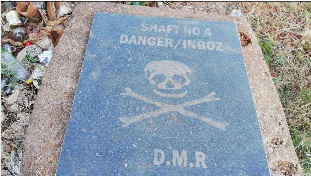
Figure 30: Granite top of rehabilitated shaft No 4.
