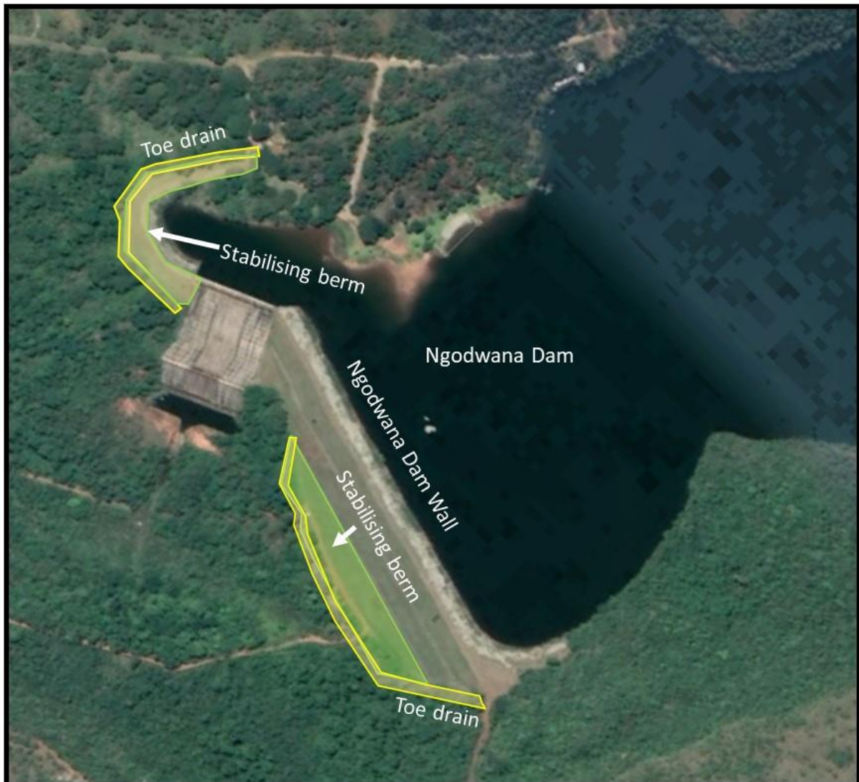
Figure 37: Dam wall berm and toe drain to be stabilised.
