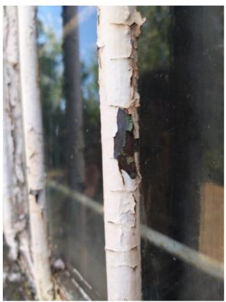
The strength of the steel bars need to be inspected, as the steel may be rusted through and need replacing. When painted all the existing paint and rust should be removed. The specification can then be followed, bearing in mind that any uneveness in the surface of the steel will be visible once painted.
