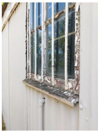
Existing timber frames in sound condition, should be stripped of existing paint either by the prescribed dry method, or paint stripper method. Once cleaned, they can receive a full coat of wood primer, similar to the new timber specification.
