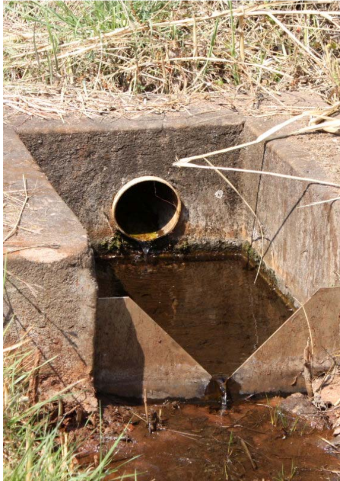
Plate G6. V-notch for Toe Drain East and West.
