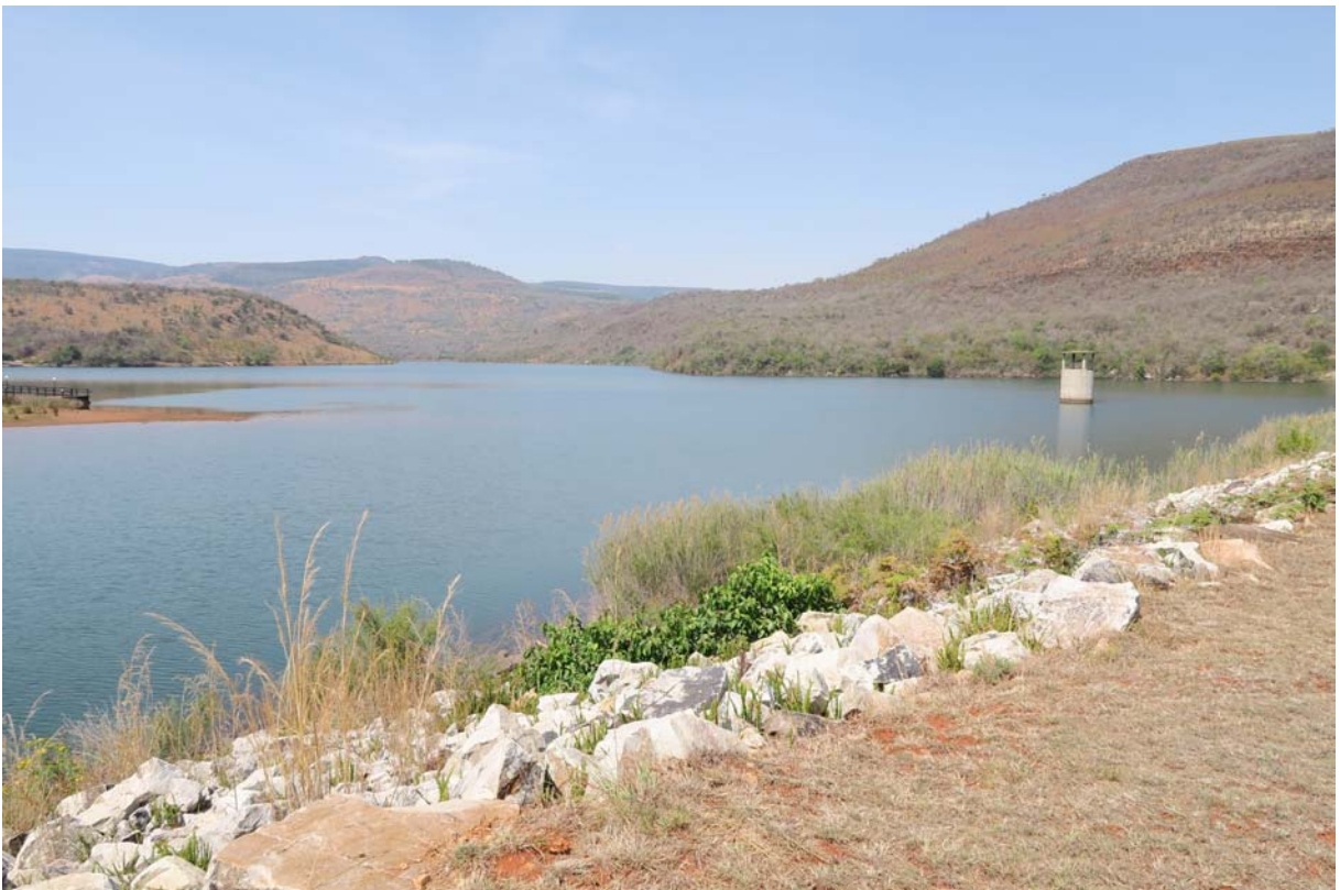
PLATE 12:- Dam basin and intake tower
