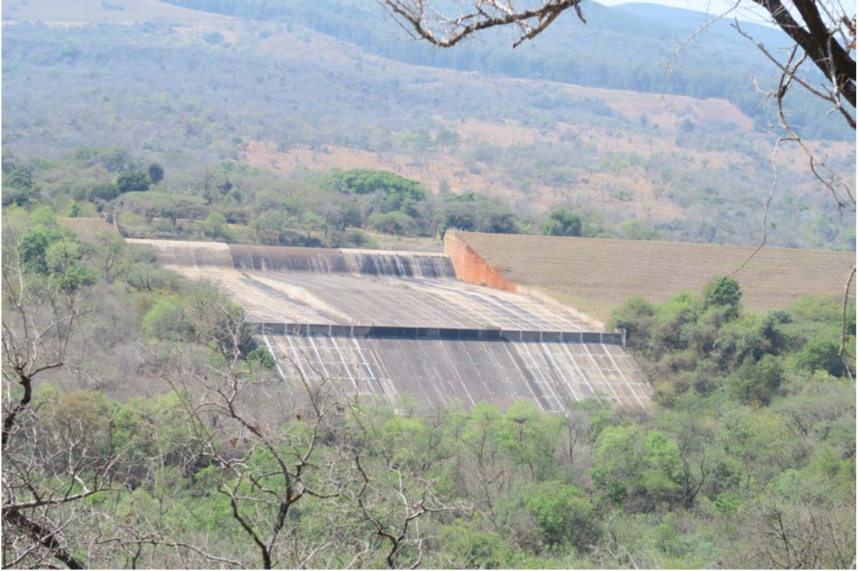
PLATE 1:- Ngodwana Dam spillway and dam wall viewed from downstream
