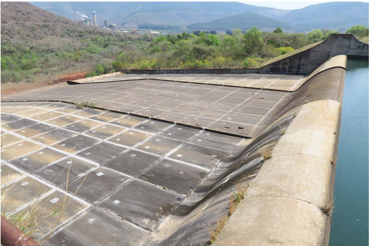
PLATE 8:- Spillway OGEE control structure and return channel
