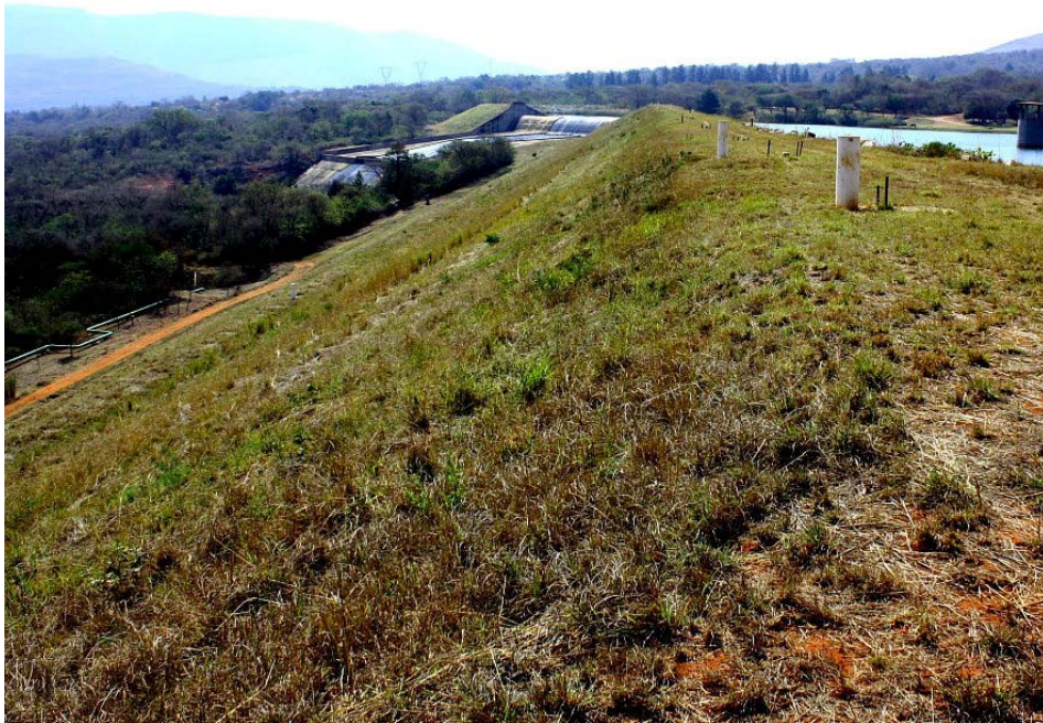
Plate G1. View of dam wall from left abutment.
