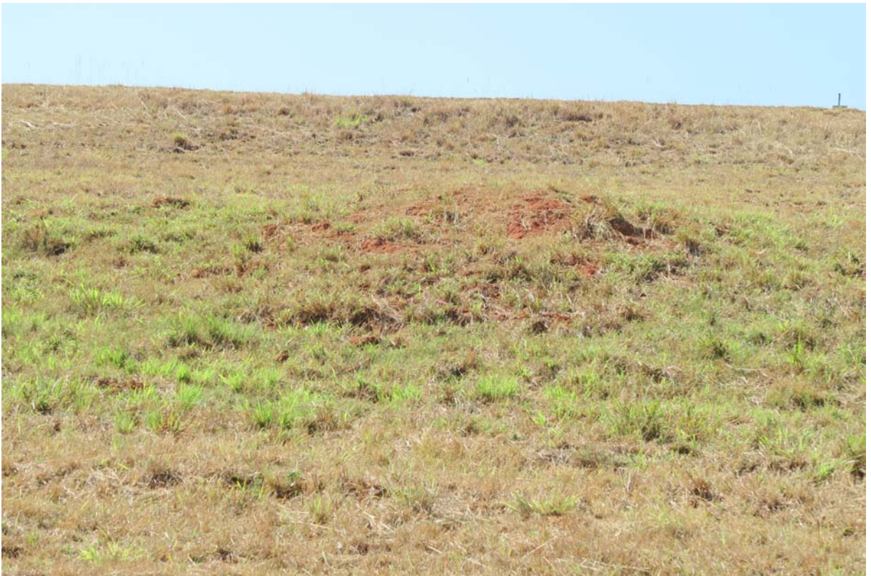
PLATE 10:- Termite nest (now dormant) on riverbed section SP4-7
