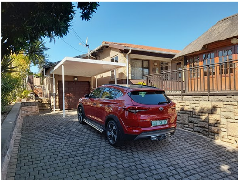
119 Doble road view from the Driveway. What is noteworthy is how neat the property is, the owners take great pride in 119 Doble road. Basic timber balustrade, with the same stone cladding tile that was seen around the front columns. Grey driveway paving is fairly new. Aluminium windows with a bespoke garage door. A simple steelwork assembly roof is present. With that being said, there is still nothing architecturally significant. Image taken 2nd of June 2022
