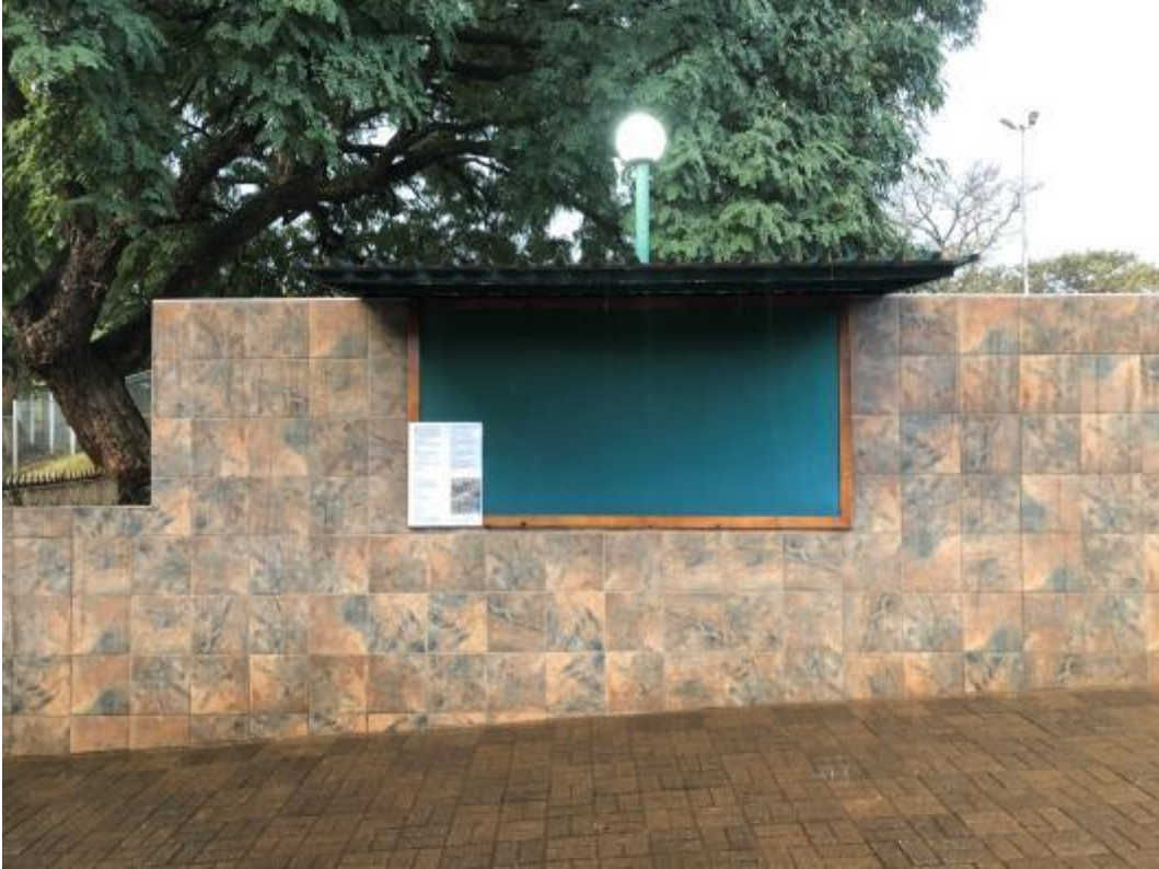
Photo 1: Notice at the notice board of the Ngodwana Shopping Centre.
