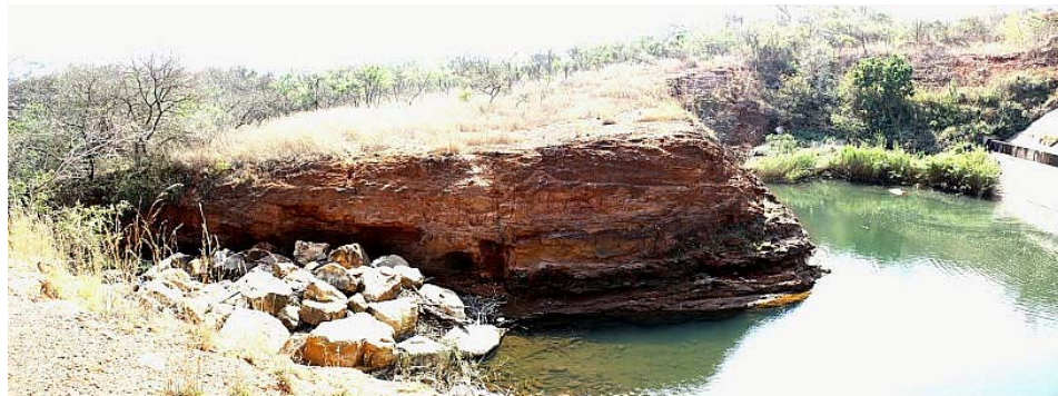
Plate G10. Plunge pool. Note erosion between rock blocks and side of channel.
