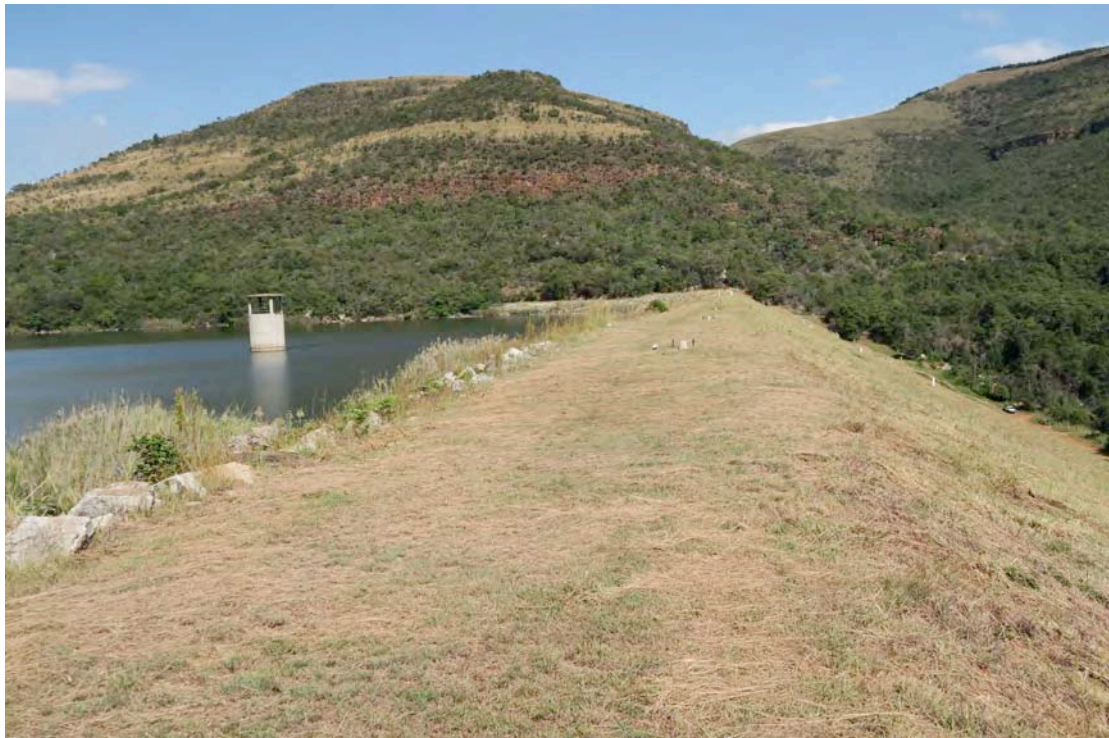
Plate 12:- Dry intake tower and embankment crest viewed from right bank / spillway (2016-05-10)
