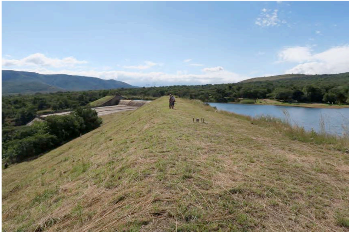
Plate 13:- Survey beacons on crest of dam wall, viewed from left flank (2016-05-10)
