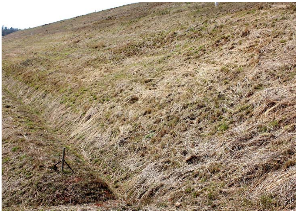
Plate G4. “Wet” area on downstream face also showing left flank (west) surface drain.
