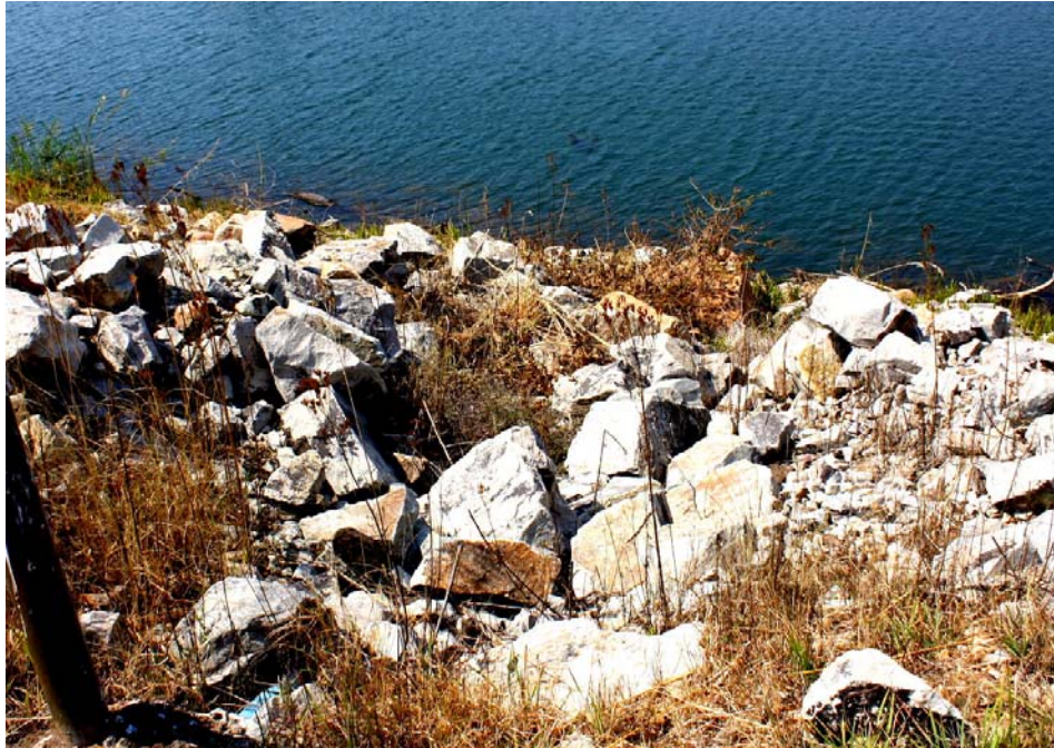
Plate G3. Trench on upstream face.
