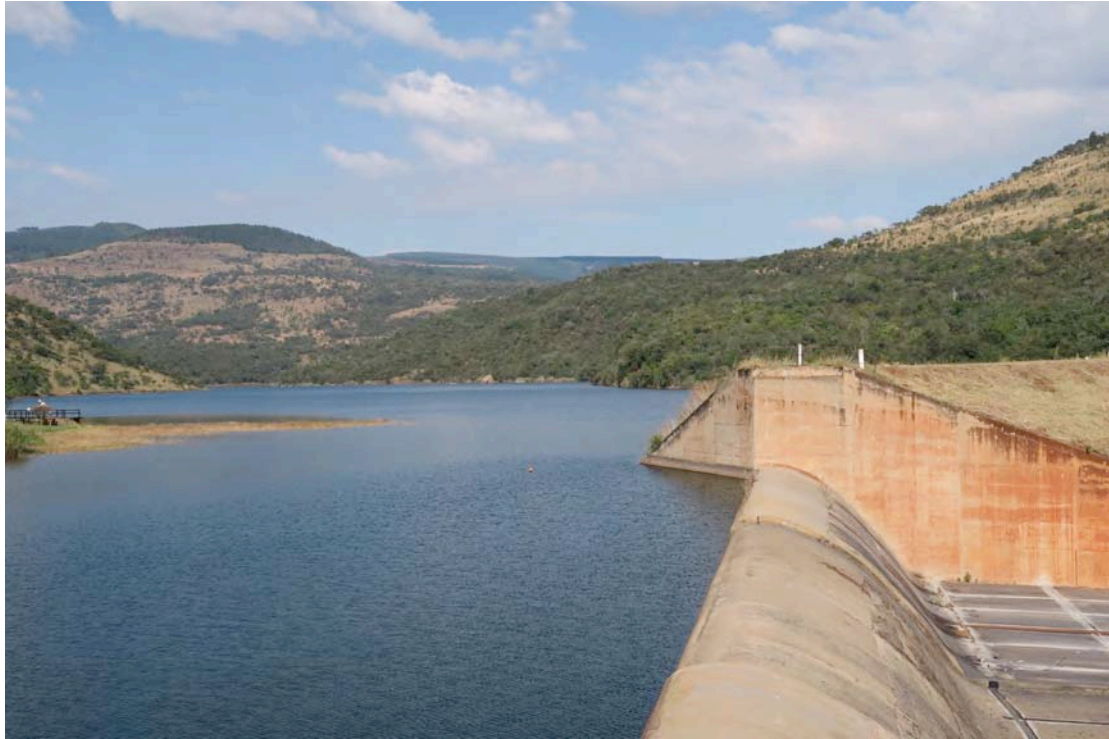
Plate 9:- Service spillway OGEE control structure (2016-05-10)
