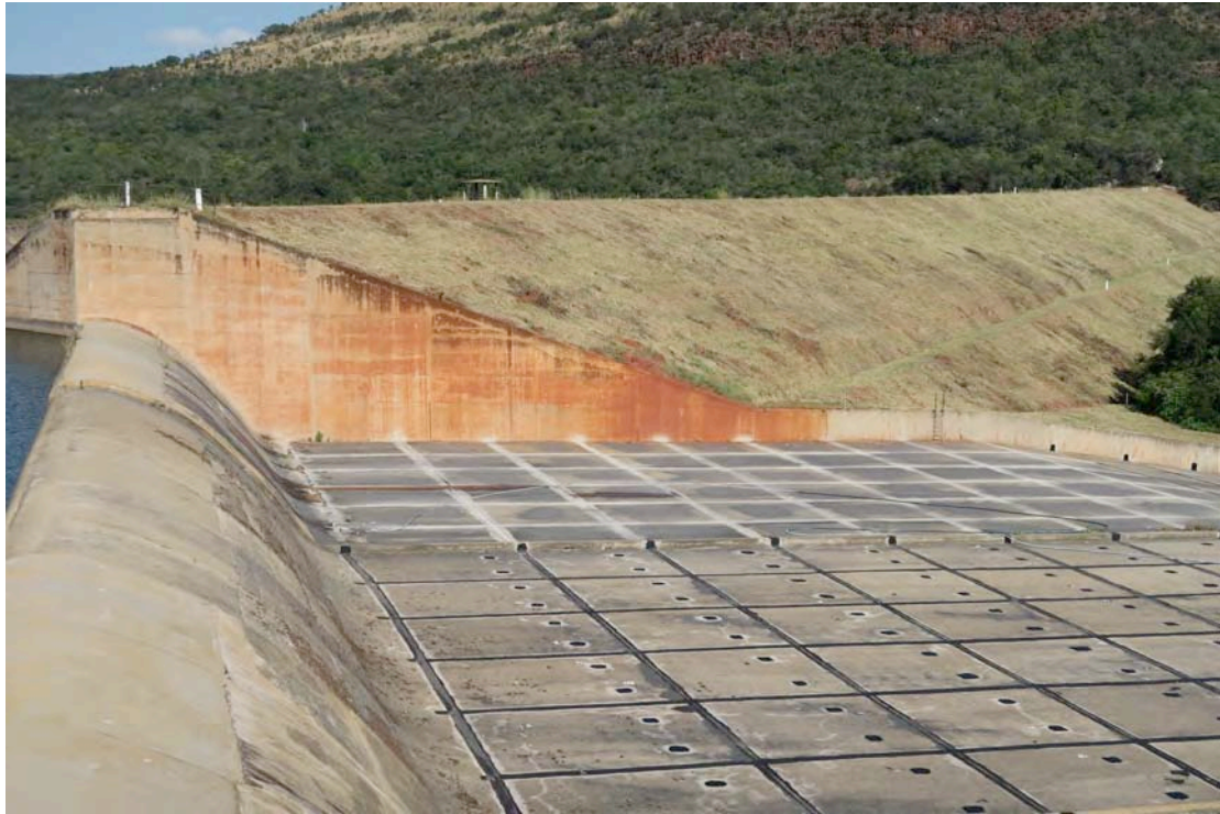
Plate 7:- View from right bank emergency breaching section across service spillway in foreground (2016-05-10)
