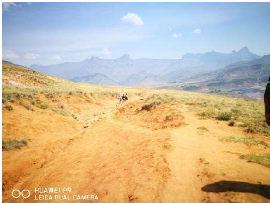
Figure 4: a portion of Qhozo access road to be constructed.
