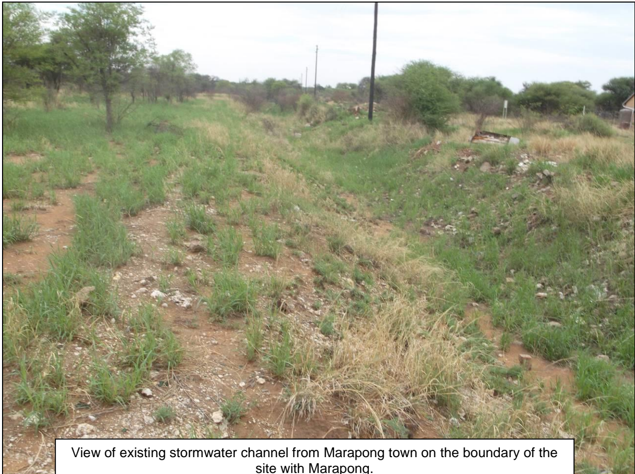
View of old evaporation dams on the southern part of the site. The area will be levelled and used as Business erven.
