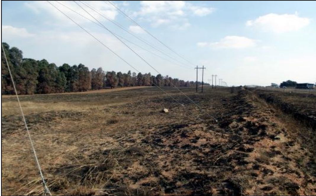
Fig. 7. Site KSO C. Looking towards the west across the razor wire fence into the proposed servitude area of the substation. An estimate is that no heritage resources are located here.
