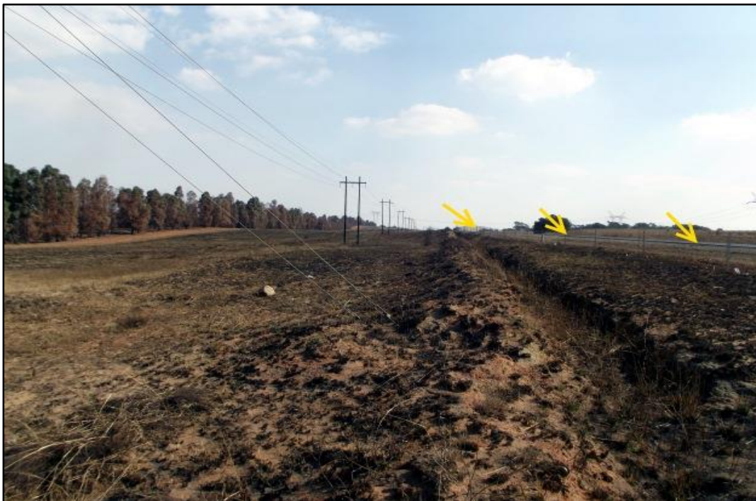
Fig. 8. Site KSO C. Looking towards the west. The servitude of the proposed substation runs along the road and trees visible from the left corner of the photo. Access to this area was not granted. Yellow arrows indicate the razor wire fence.
