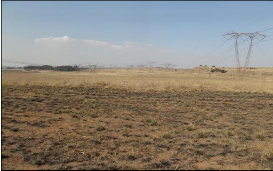
Fig. 3. Site KSO A. Looking towards the south. This is the location of the proposed new substation.
