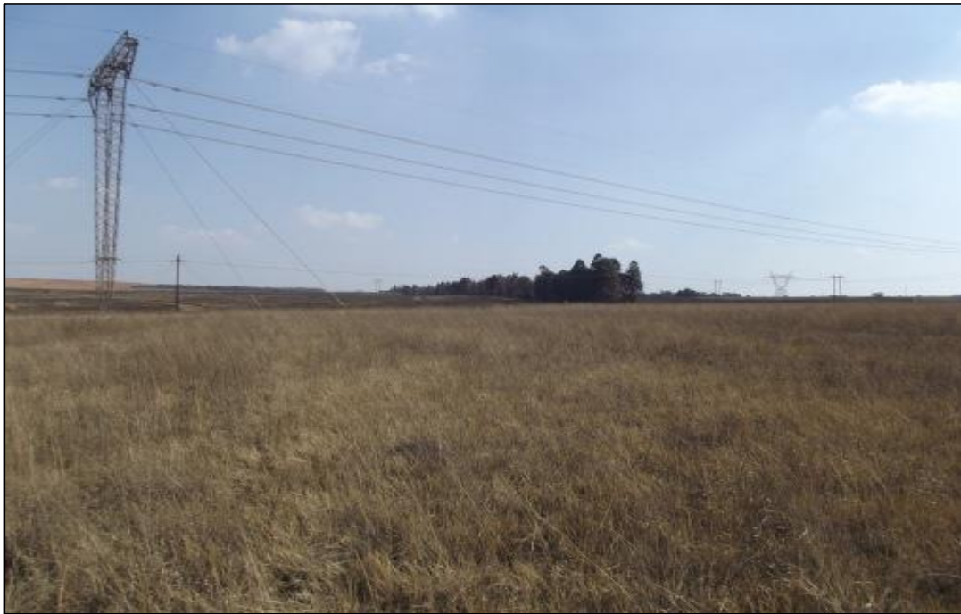
Fig. 4. Site KSO B. Looking west, in the vicinity of the proposed new substation.
