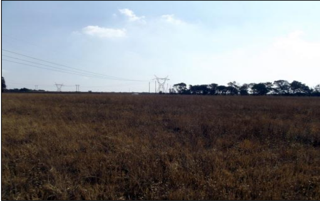
Fig. 5. Site KSO B. Looking north-west. The proposed new substation will be located in this area.
