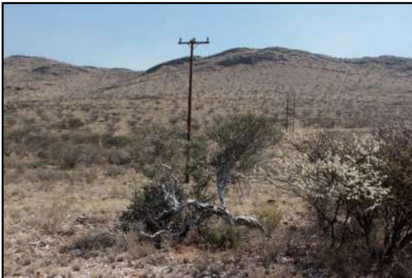
Figure 22. The Eskom power-line with old Boscia albitrunca tree in the foreground. These trees must be avoided since they are protected.
