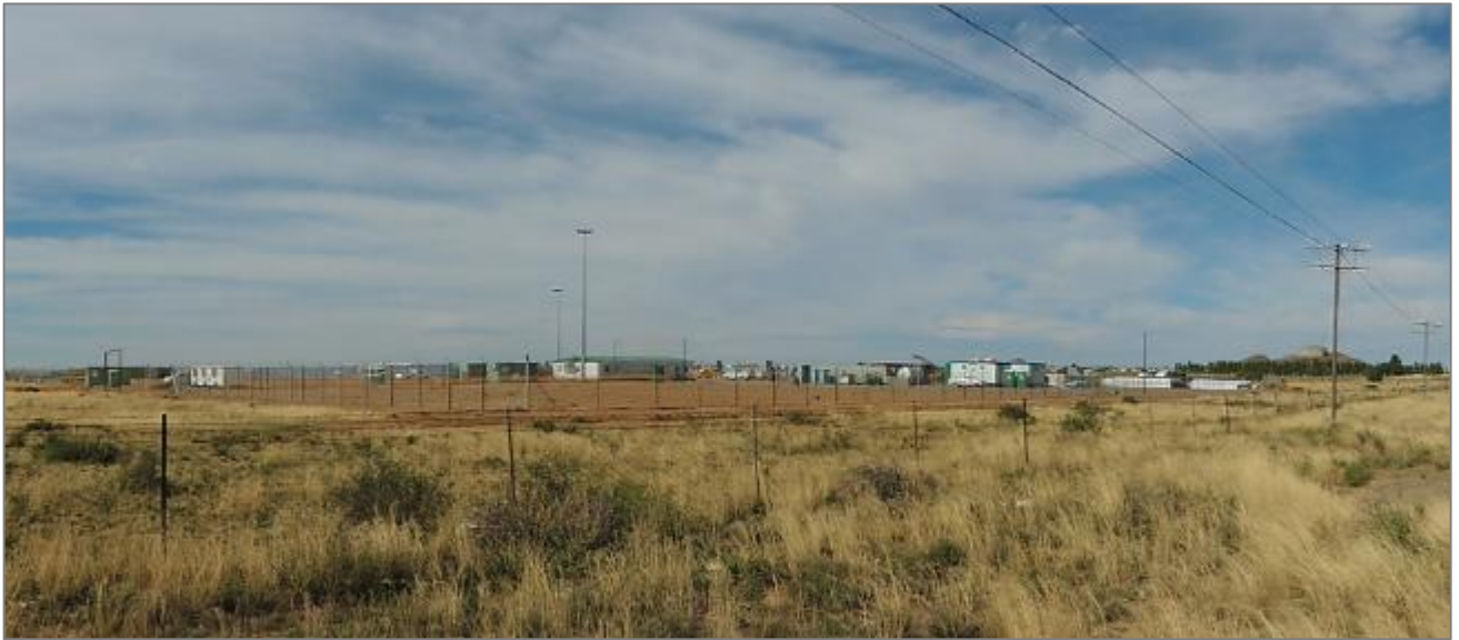
Typical construction site and laydown with fences (overhead lighting not included) (Source: VRMA)
