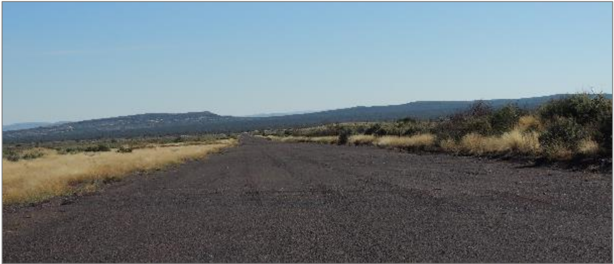
Figure 13: Photograph depicting the abandoned iron ore mine haul road
