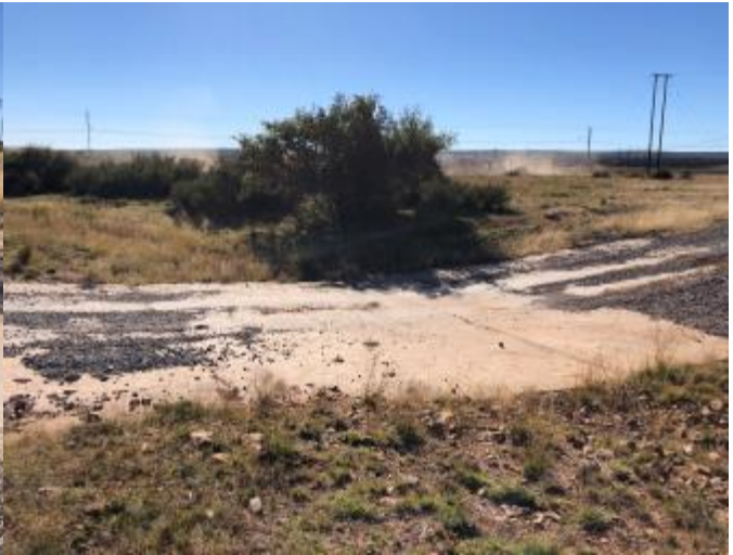
Plate 4: Upstream view of Concrete Drift
