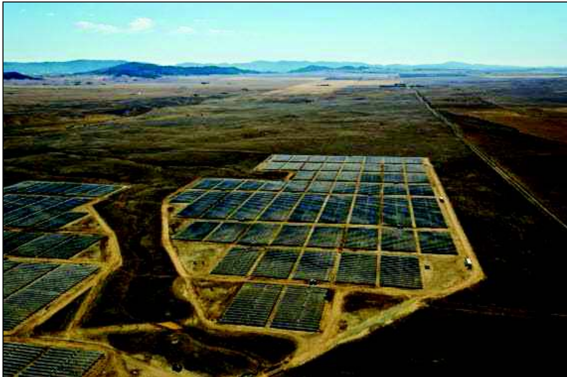
Figure 1: Example of a PV facility in a landscape similar to De Aar (image courtesy of Mulilo, cited in Aurecon, 2013 ).
