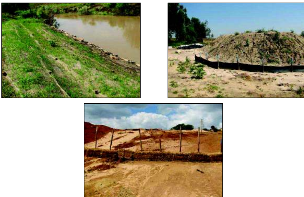
Figure 25: Typical soil erosion mitigatory measure: BioJute Installation ( top left ); a silt fence protecting a stockpile ( top right ) and pegged hay bale wall used to reduce runoff velocities ( bottom )
