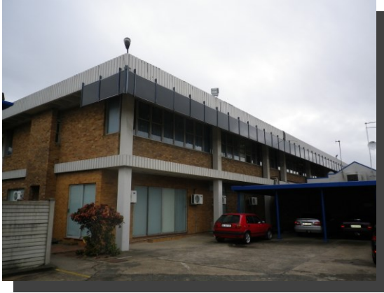
Building 26: Southern View:
