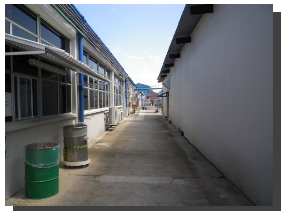
Building 4: North Eastern View:
