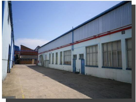
Building 10B: North Eastern View:
