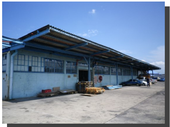
Building 10A: North Western View:
