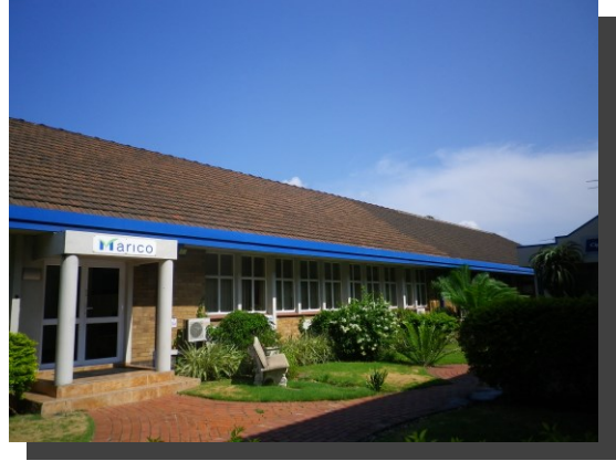
Building 25: Northern View:
