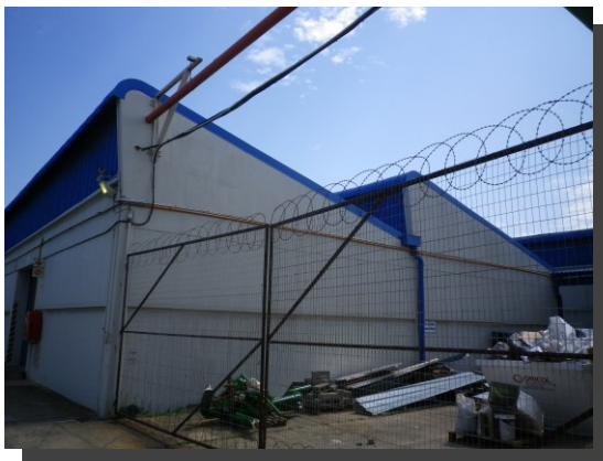
Building 6: North Eastern View:
