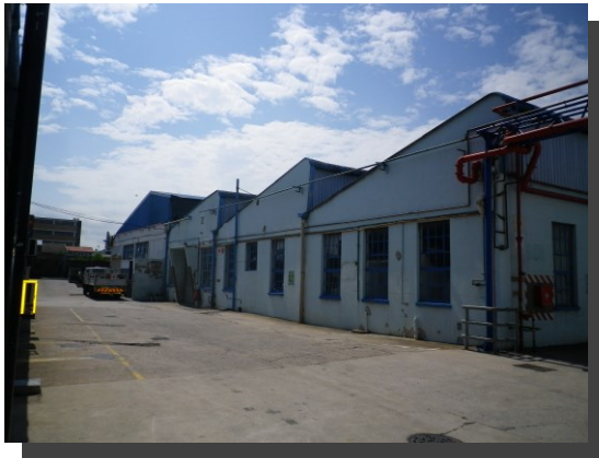
Building 10B: Southern View:
