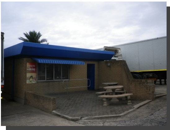
Kiosk Building: Northern View:
