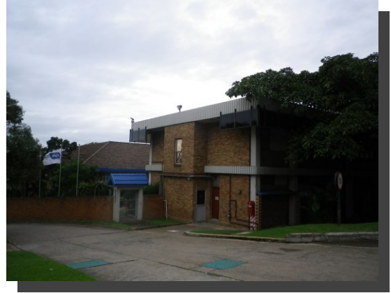
Building 26: Northern View:
