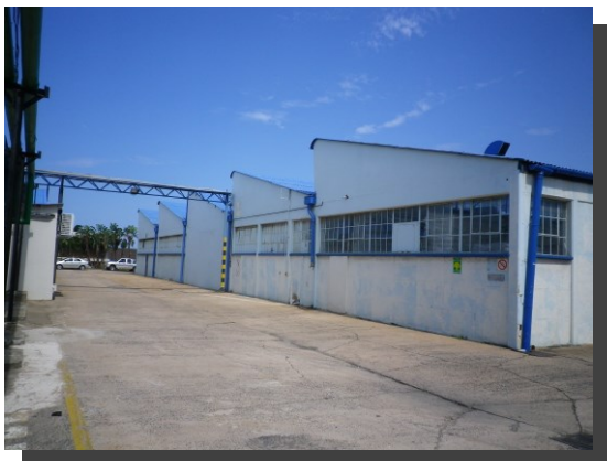
Building 3: North Eastern View:
