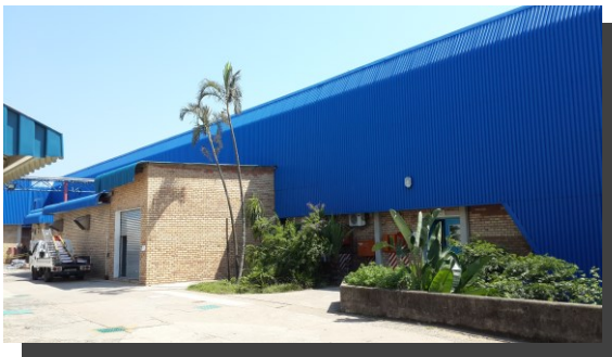
Pharmaceutical Building: South View:
