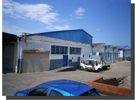
Building 10A: South Western View:
