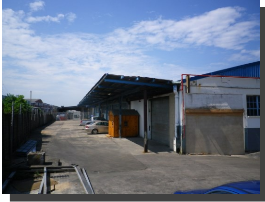
Building 10A: Western View:
