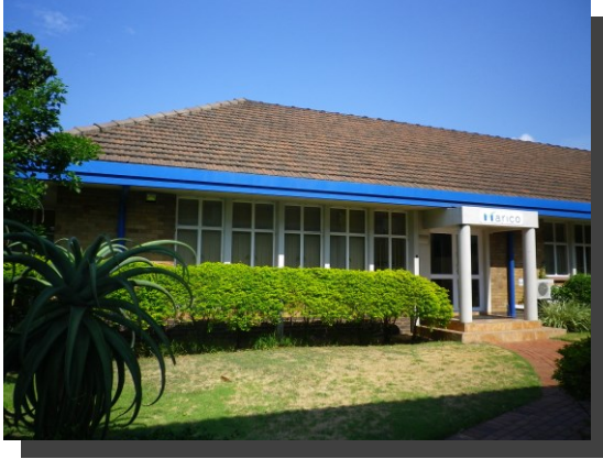
Building 25: Northern View:
