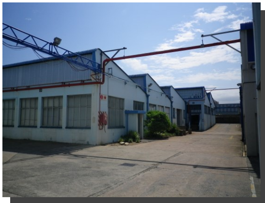
Building 10B: Eastern View:
