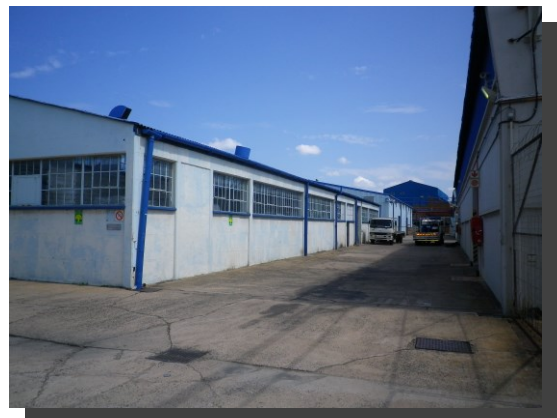
Building 3: Northern View:
