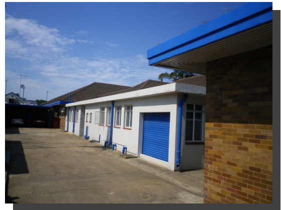
Building 25: South Western View:
