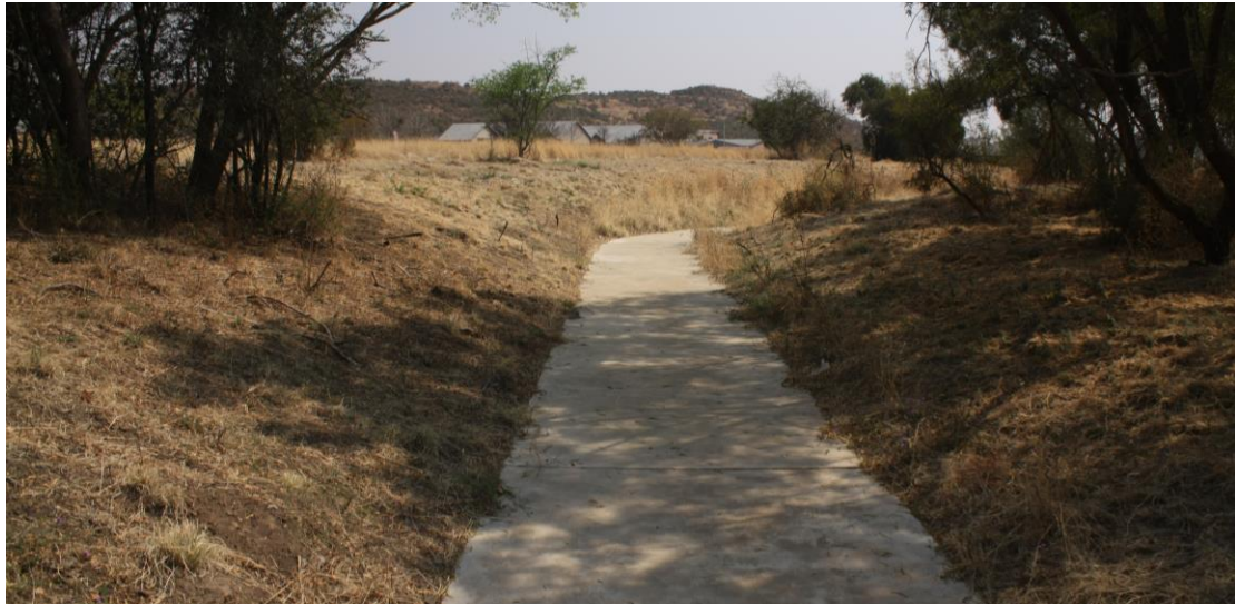
Figure 9: View of the drainage line downstream of the site where it has been canalised. It is recommended that the proposed development incorporate it in much the same manner.
