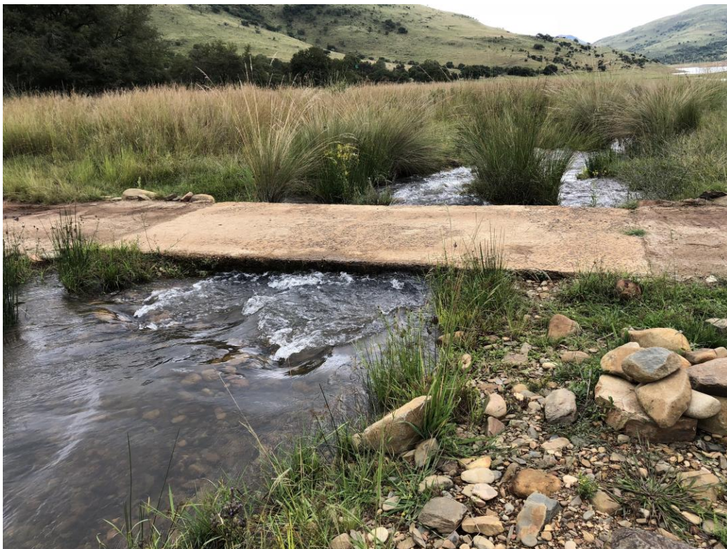
A TYPICAL CAUSEWAY PIPE CULVERT COMBINATION
