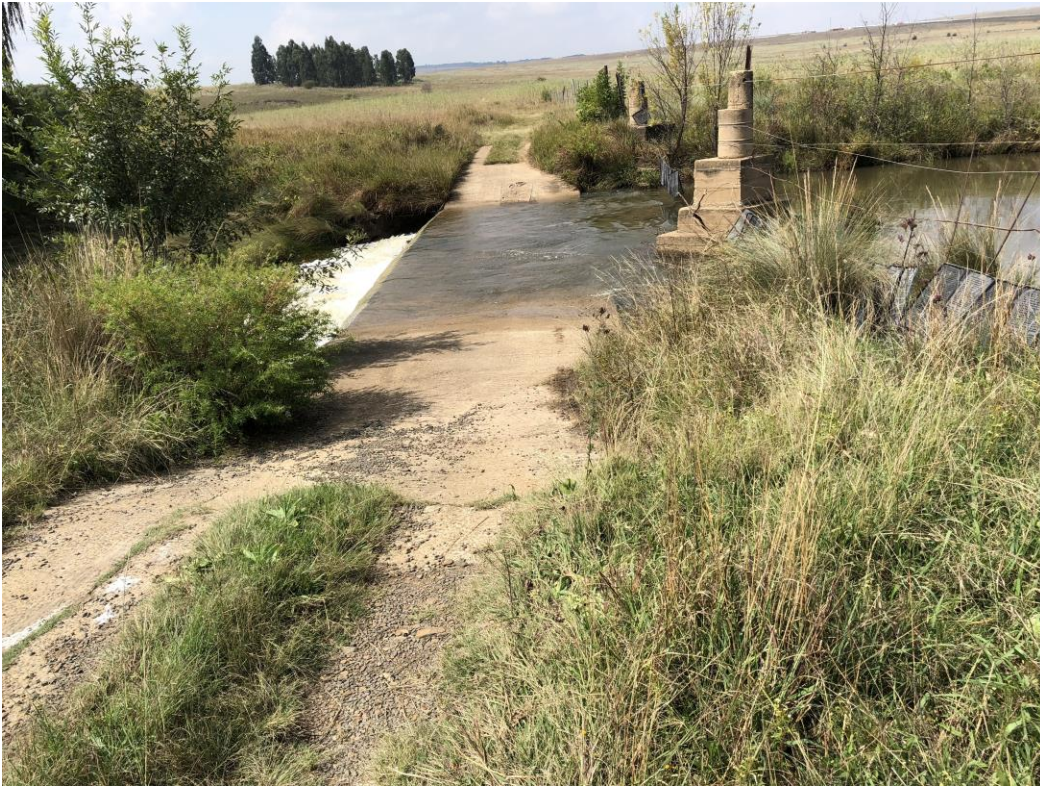
A CONCRETE CAUSEWAY ON IMPORTED ROCKFILL
