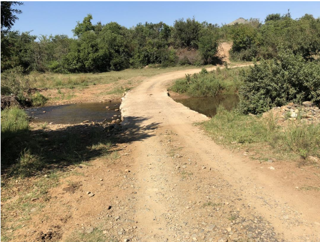
CAUSEWAY WITH PIPE CULVERTS
