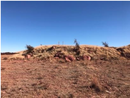
Figure 22: Soil and rock dumping within the eastern proposed soil stockpile and parkup area (facing west).
