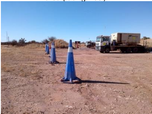
Figure 24: Cleared area within the eastern proposed soil stockpile location.
