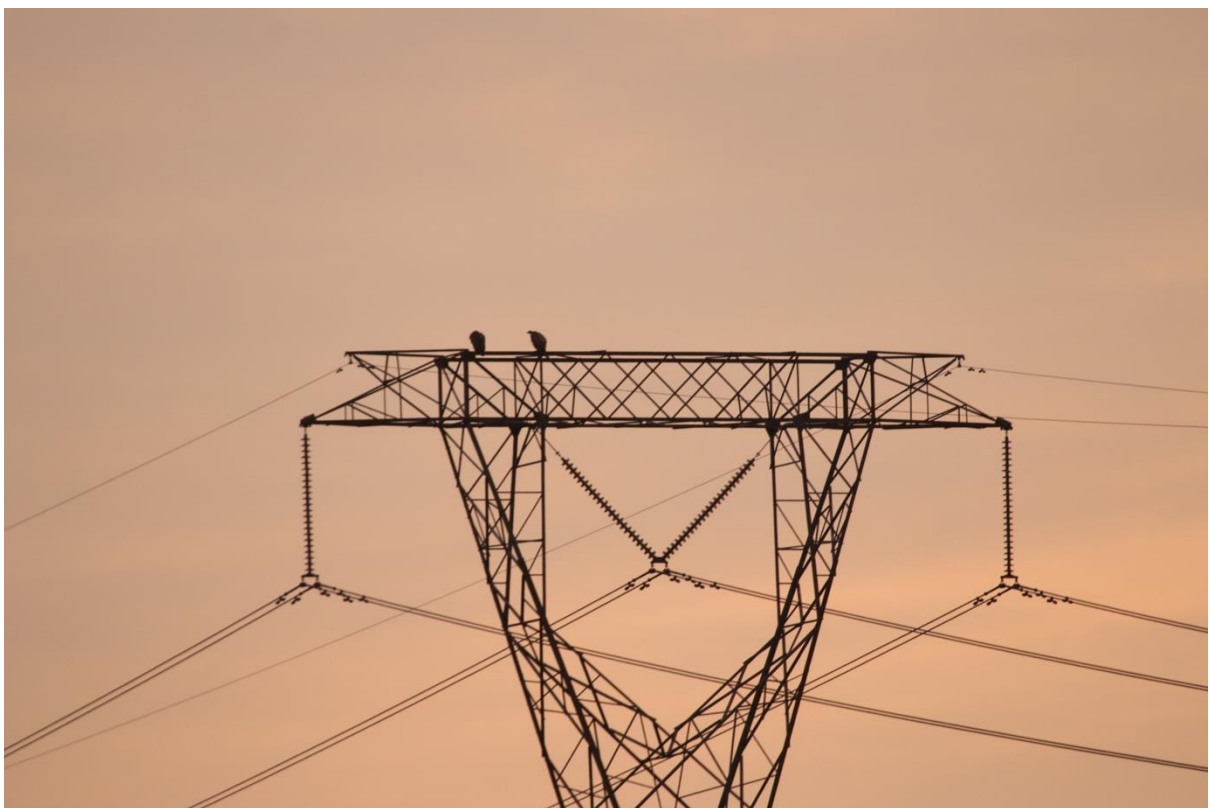
Figure 34. Two Cape Vultures ( Gyps coprotheres ) roosting on overhead transmission lines.
