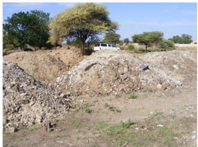
Figure 24: Boschfontein Spruit – Signs of the road and bridge construction activities.
