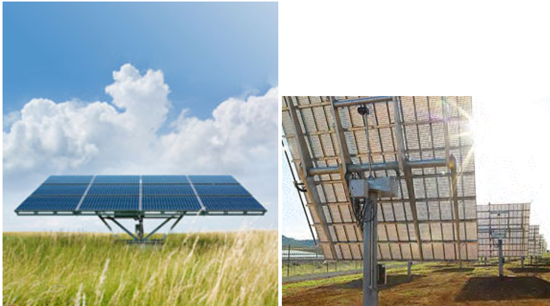
Figure 4a: Example of Solar Panel Free Standing dual axis.(source Apsolutions)
