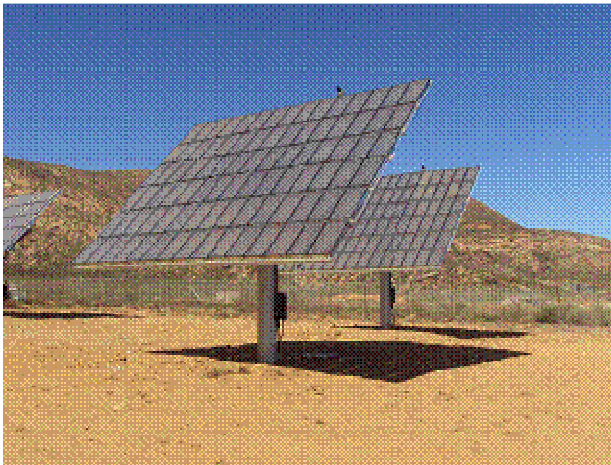
Figure 4c Example of Solar Panel Free Standing dual axis with CPV technology
