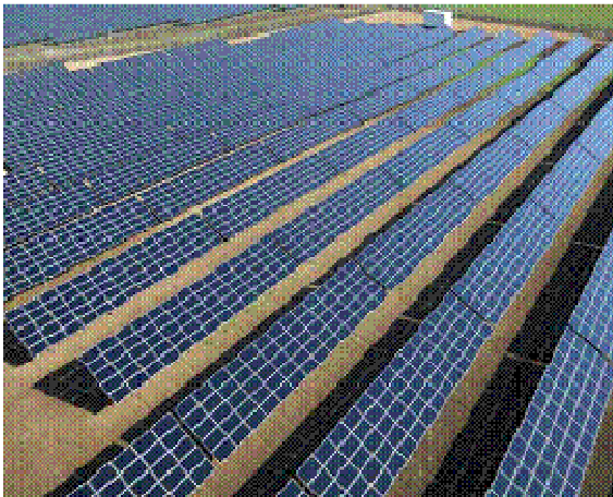
Figure 5: Example of Fixed Tilt Single Axis tracking Table Installation
