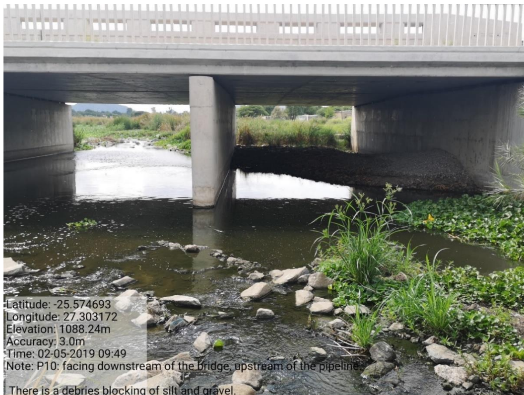
Photograph 6-1: A bridge located upstream of the proposed Bospoort pipeline
