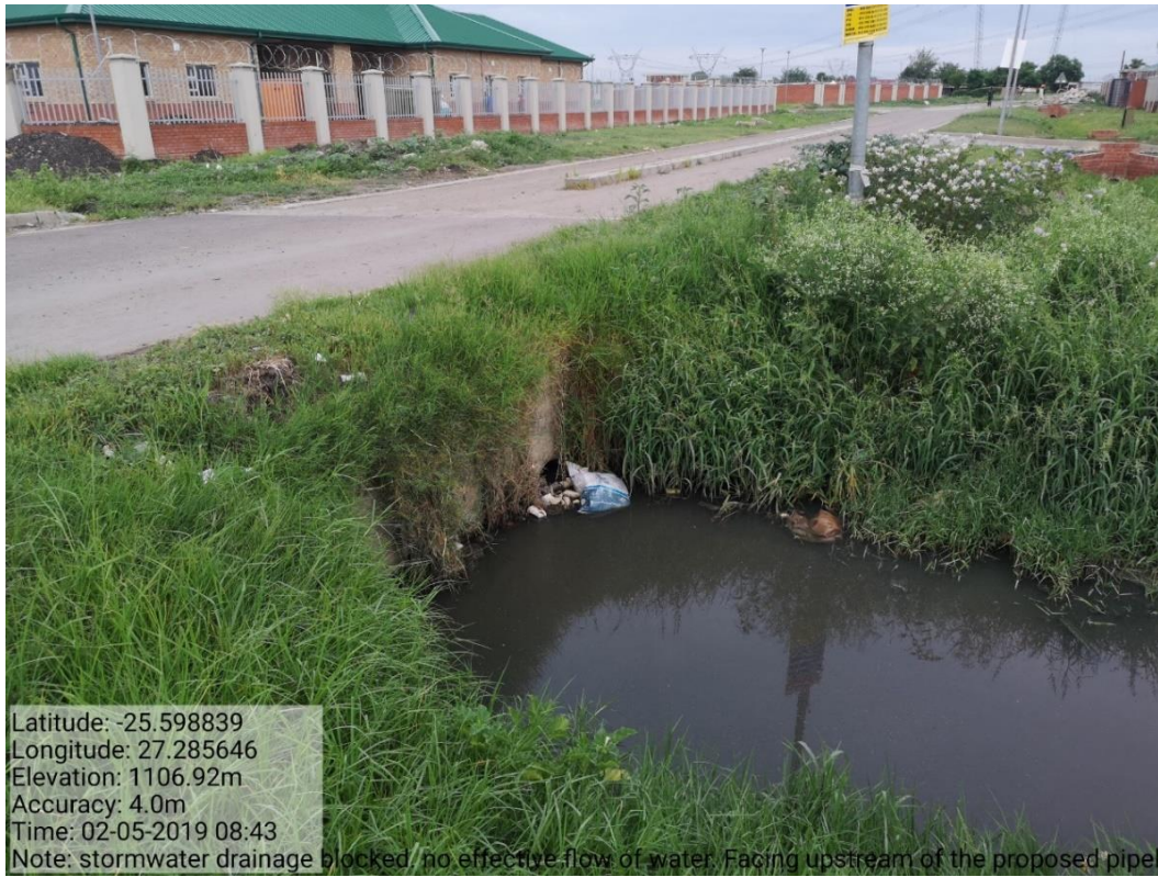
Photograph 6-2: A culvert situated upstream of the proposed Bospoort pipeline
