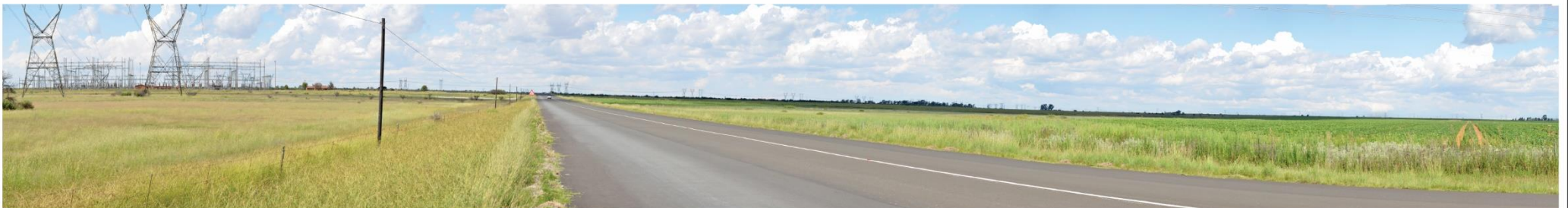
CL 263 along R730, northbound, view of the Eskom Theseus Main Transmission Substation, on the left note the existing powerlines running to the substation in the fore- and backgrounds. The project powerline will run in the same corridor as the existing powerlines in the background.
