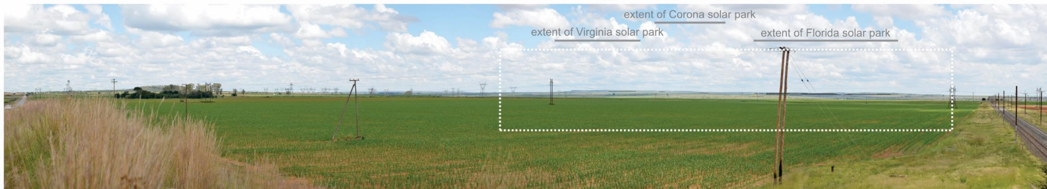
CL 207 photomontage: Virginia solar park at approximately 16,5km, Corona solar park at approximately 11,8km and Florida solar park at approximately 8,8km
