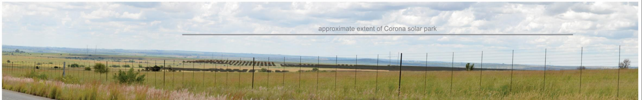
CL 249 zoomed in area, solar park components partially hidden by topography
