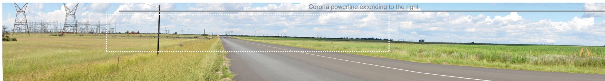
CL 263 photomontage of Corona powerline approximately 900m from this view point following in the corridor of the existing powerlines.
