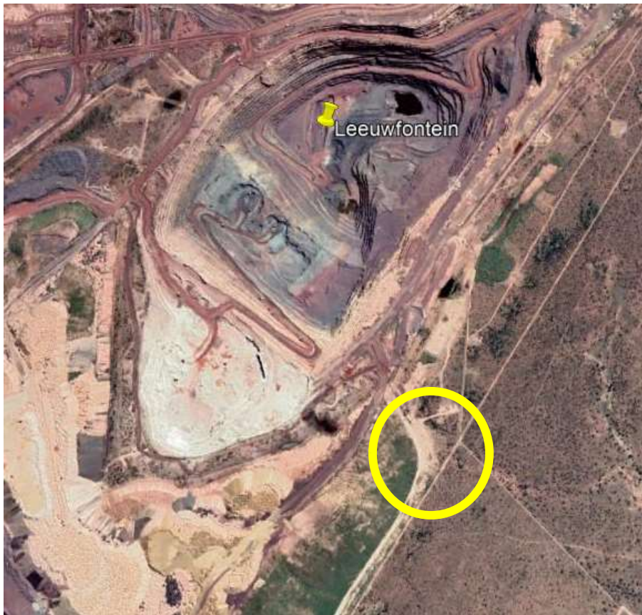
Figure 53: Location of sediment problem at leeuwfontein pit
