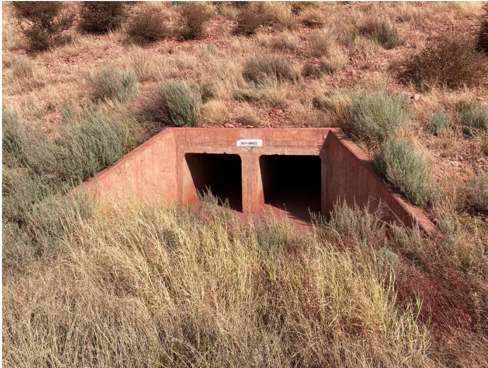
Figure 27 : Rail loop culvert
