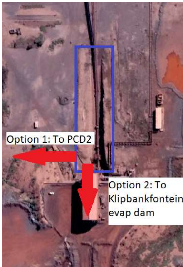
Figure 25: New bund walls around incline shaft and proposed pumping options
