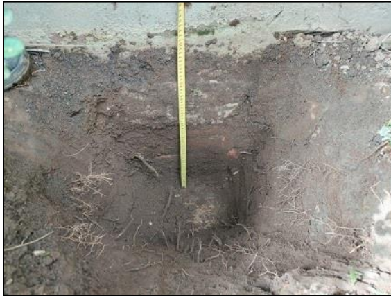
Plates 20 & 21: TP W1 & TP W2 showing the foundations measured at the existing workshop area
