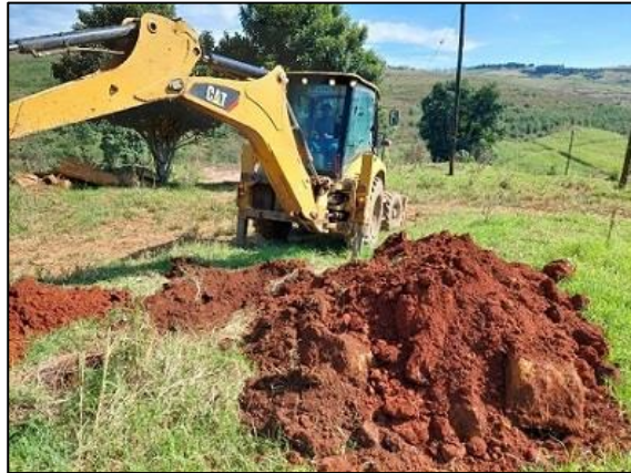
Plates 22 & 23: Colluvium overlying residual dolerite soils comprising sandy clays with occasional dolerite and sandstone boulders
