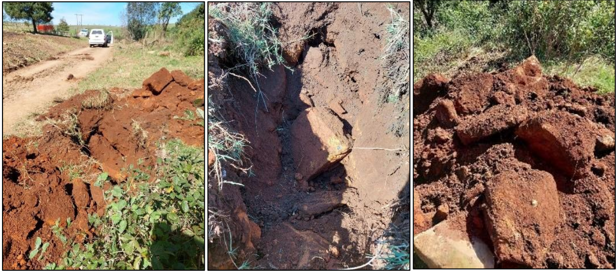
Plates 26 to 28: TP7 and TP8 excavated along the access road for the Forest Village. These test pits show abundant sandstone boulders in a matrix of clayey sand
