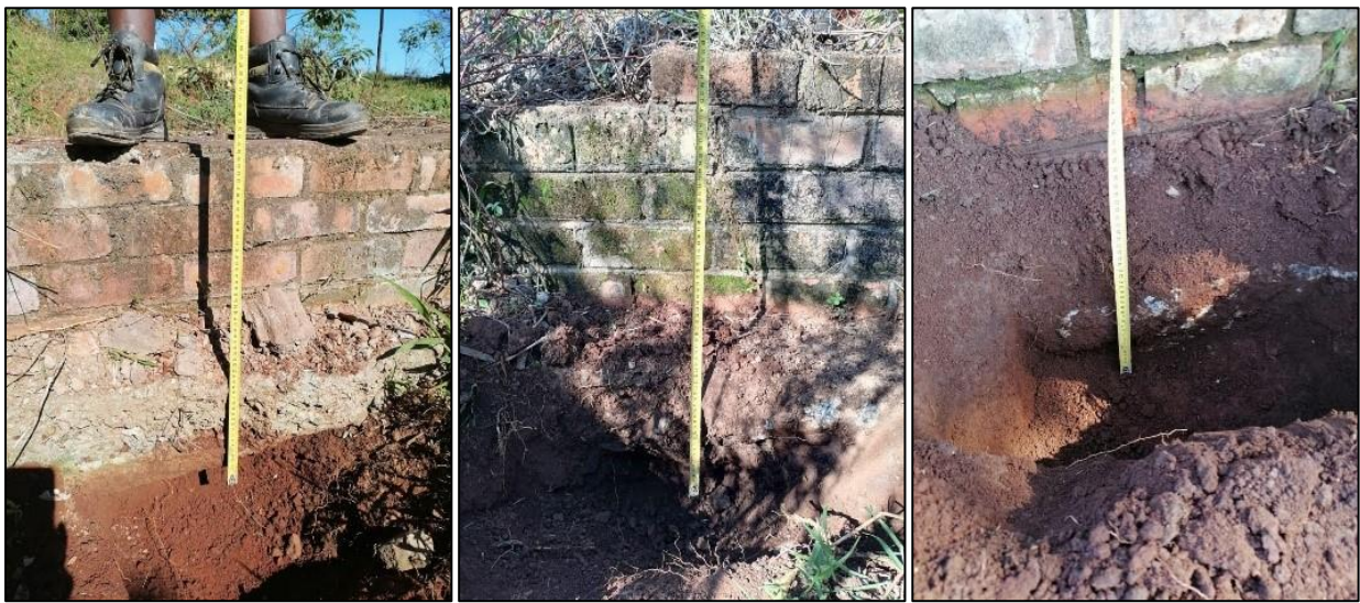
Plates 17 to 19: Foundations of partially demolished Farm Houses - Forest Village area
