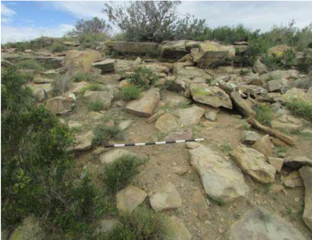
Figure 13: Collapsed stone-walled enclosure on Site 11.
