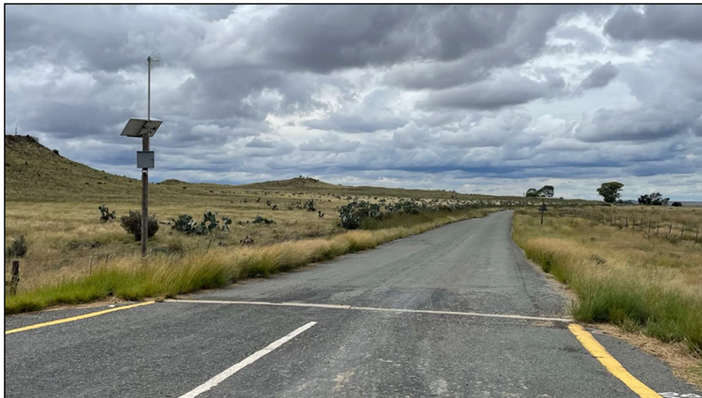
Figure 8: Burgerville Gravel Road
