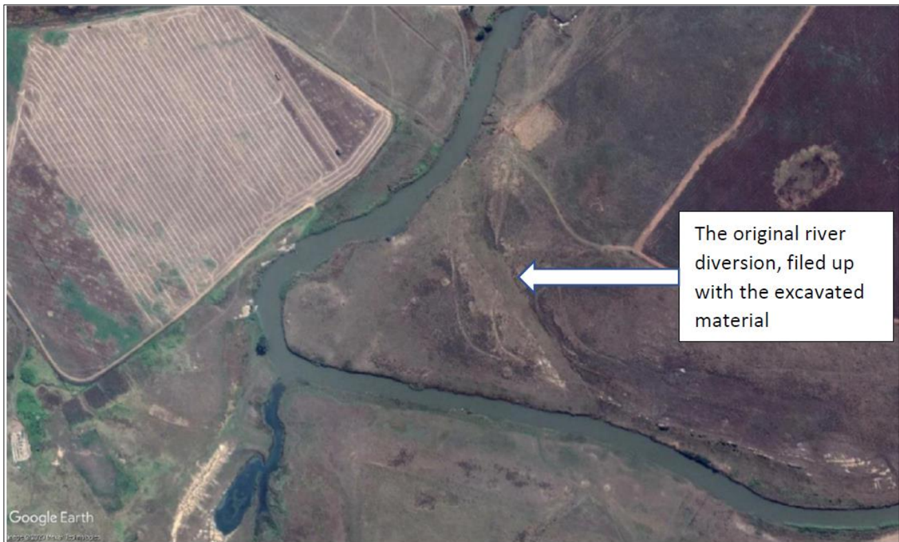
Figure 6: Original dug river diversion site
