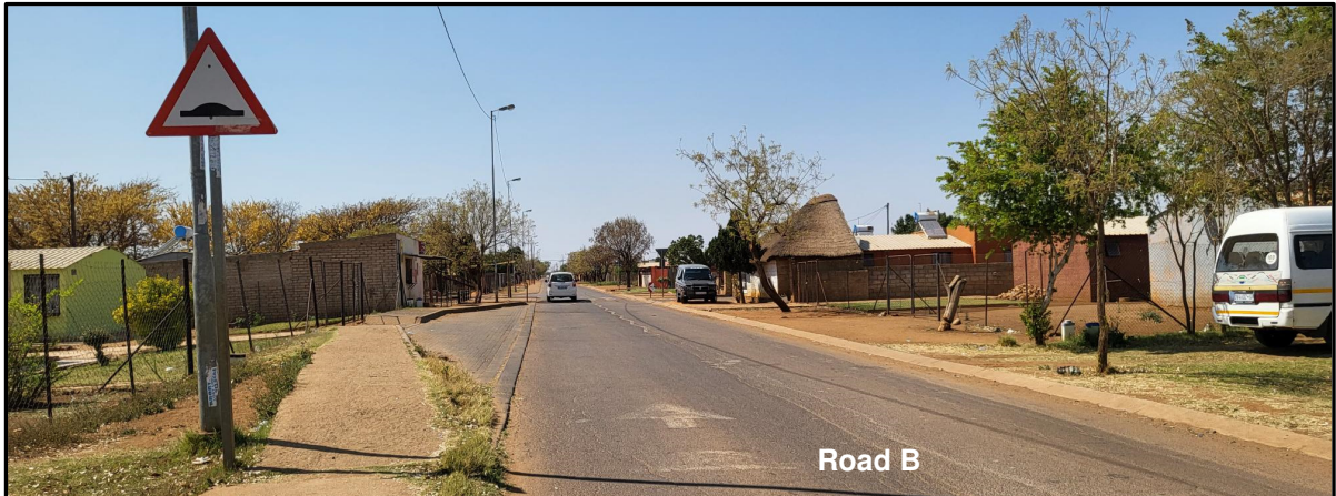
Photo 3 – Existing Minibus-taxi layby along Road B
