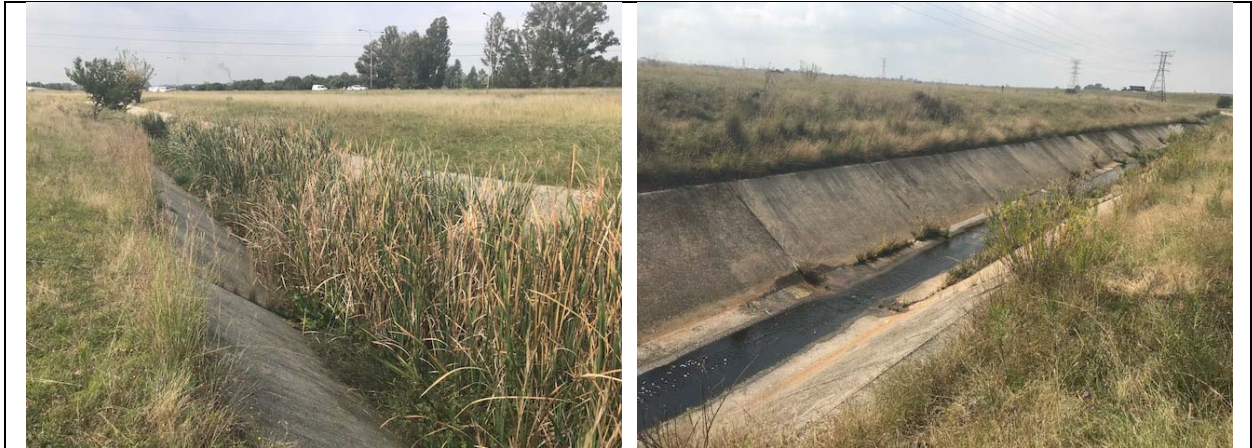
FIGURE 7: EXISTING CONCRETE LINED STORMWATER CHANNEL
